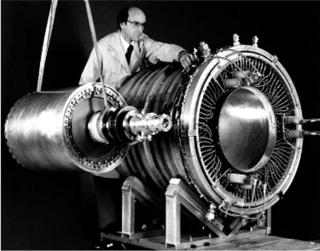
Fig. 4. General Electric 20 MW LTS generator (1981).
