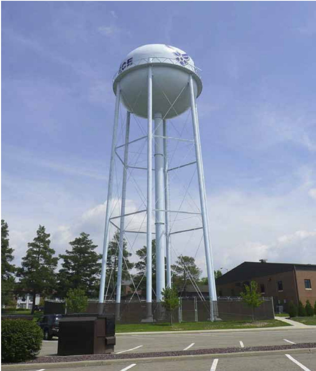
View of the water tower (CERL).
