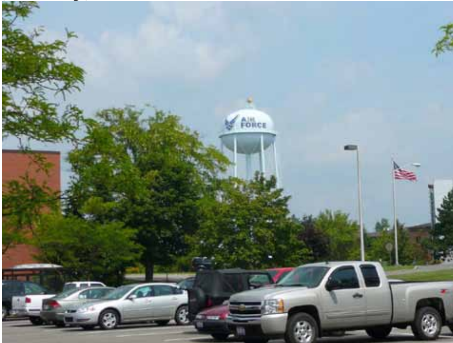
1. Oblique view of the south elevation (Building 407 – headquarters, on left)
