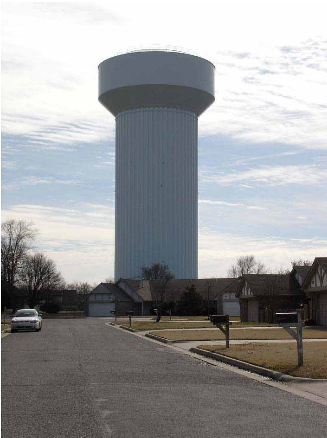
Figure 9. Hydropillar water tower in Tulsa, OK (Topato on Flickr.com).
