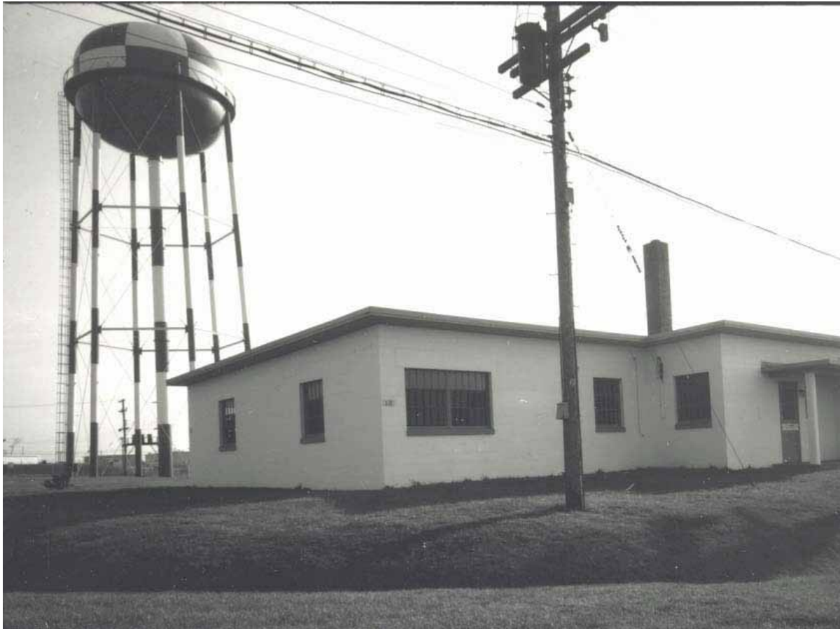
Historic photograph depicting the water tower (Source: YARS CE). The double-ellipsoidal design of the tower is known for being one of the most economical designs. The tower itself reaches a height of about 145 feet. The original checkerboard paint pattern has been replaced through several paint iterations to include the Air Force name and insignia.
