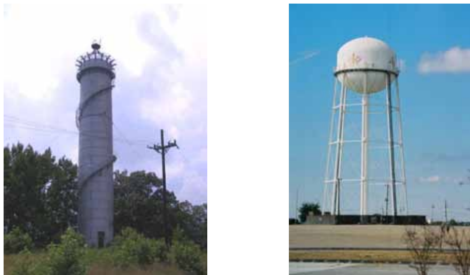
Figure 3. Standpipe at Naval Support Facility Indian Head, MD on left and an elevated water tank on right at Fort Gordon, GA (CERL).
