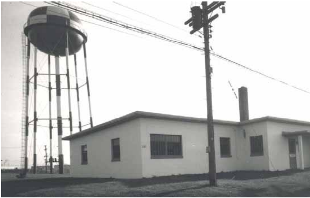
Figure 14. Two historic photographs showing the water tower (Source: YARS CE).
