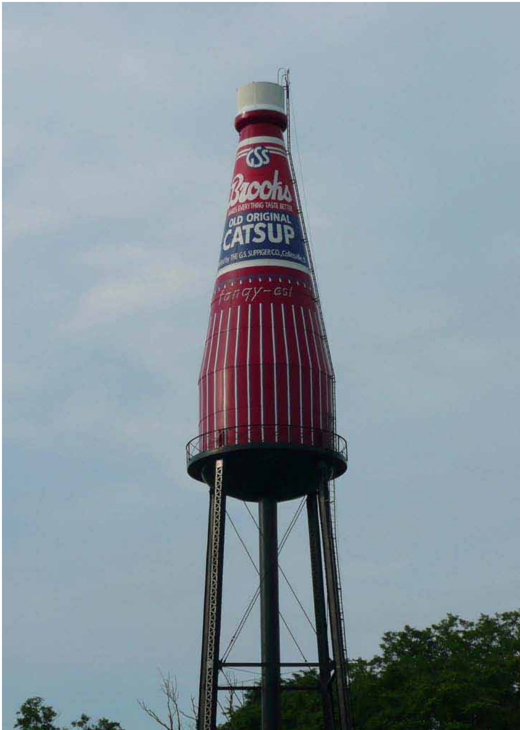
Figure 12. Collinsville, IL catsup water tower (CERL).
