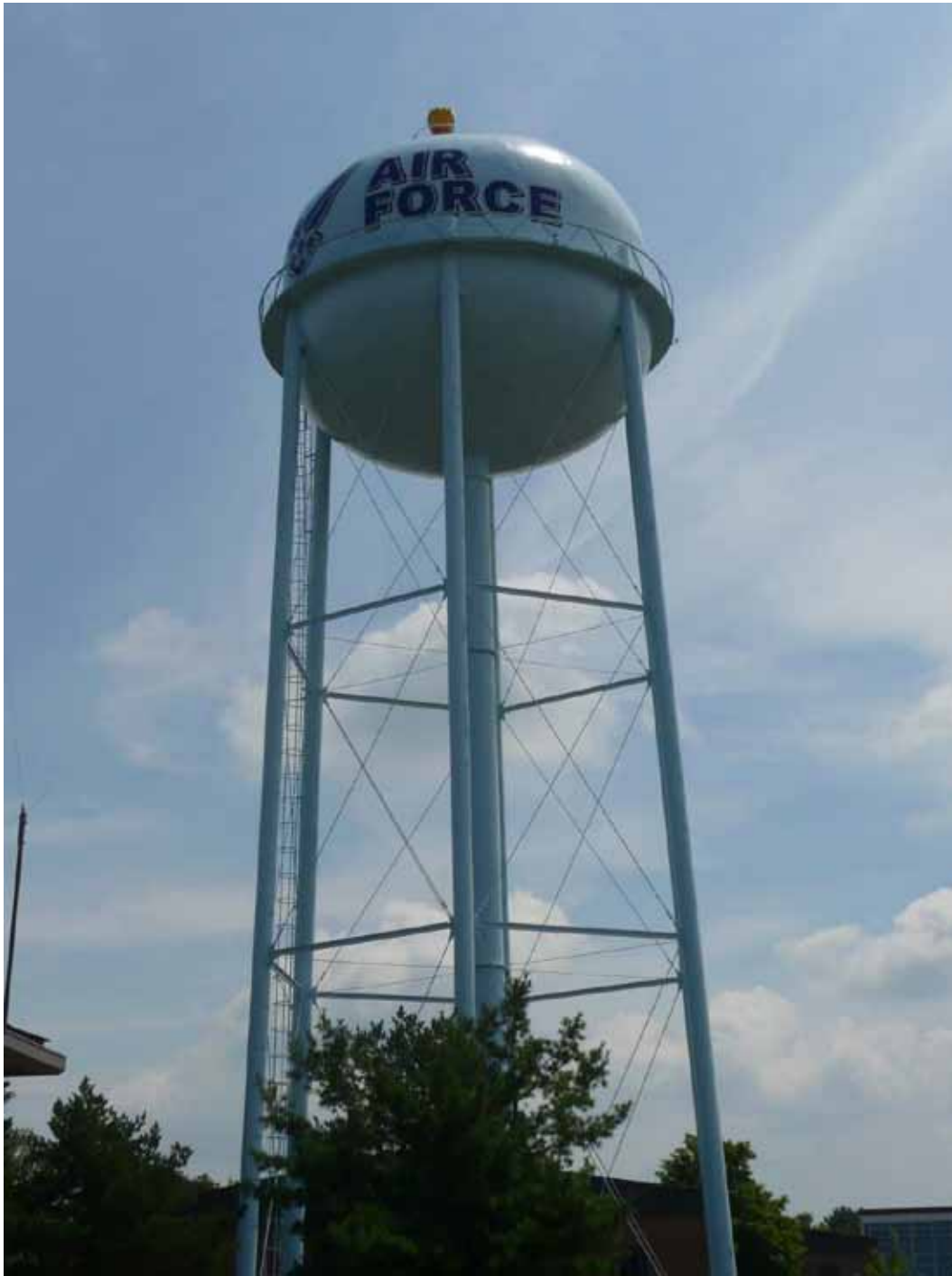
Figure 6. Double-ellipsoidal water tower at YARS (CERL).
