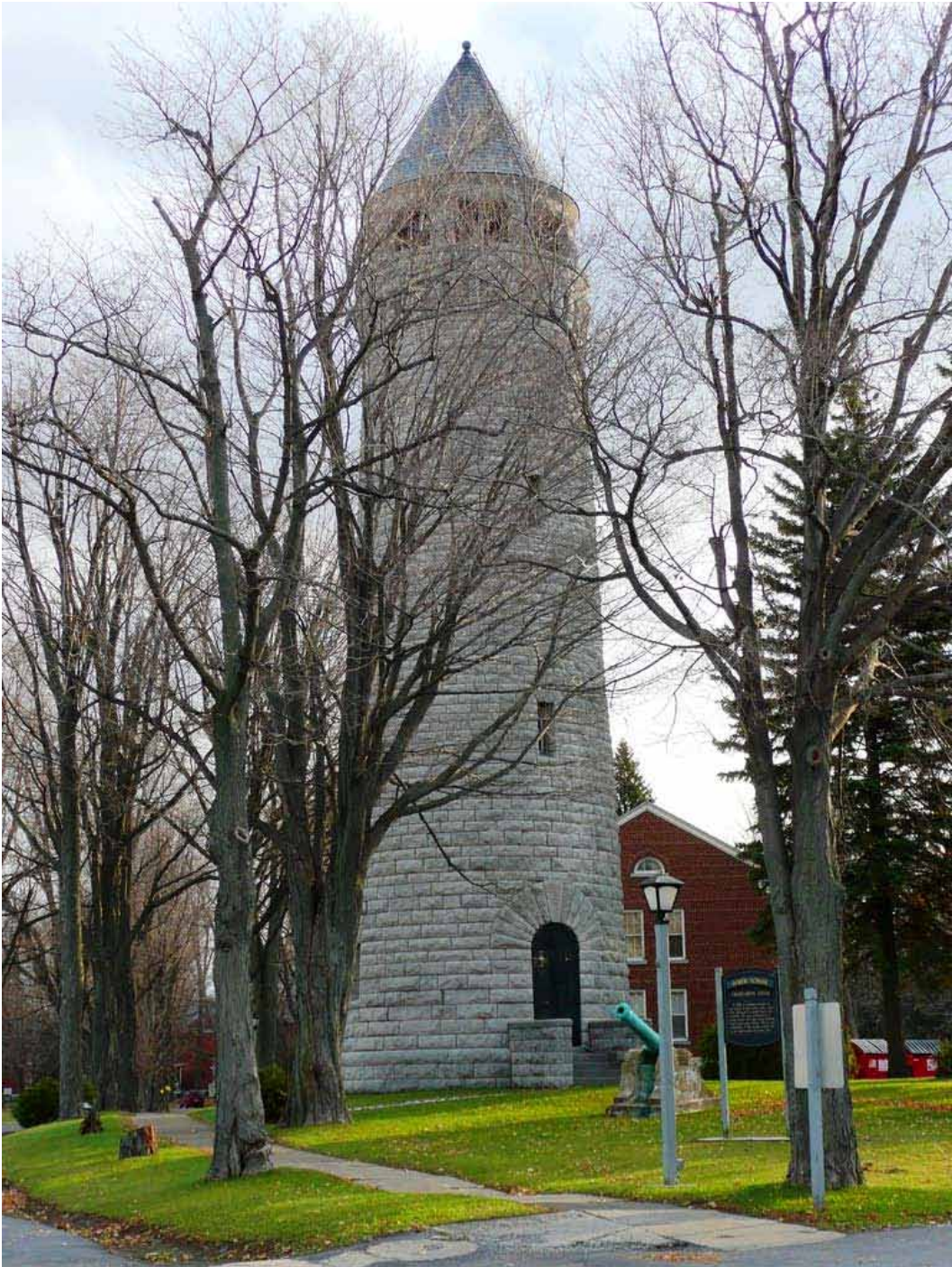
Figure 10. Madison Barracks, NY water tower (CERL).
