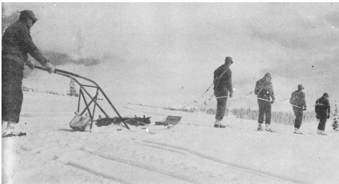
Figure 296. Members of the pack artillery on snowshoes dragging part of the 75MM pack howitzer on a sledge with special harnesses (Jay, 1948).
