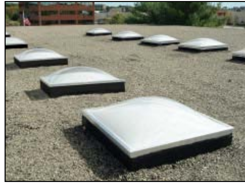
Double pane skylights with white translucent interior lens
