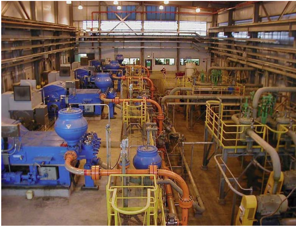
Figure 33. Antamina's mine pump station consisting of four positive displacement 1,750 hp (piston) mainline pumps (source: Pipeline Systems, Inc.).
