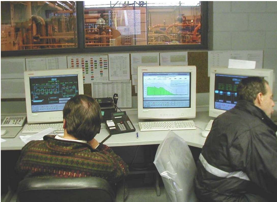
Figure 34. Antamina’s pipeline transport system control room (source: Pipeline Systems Inc.).
