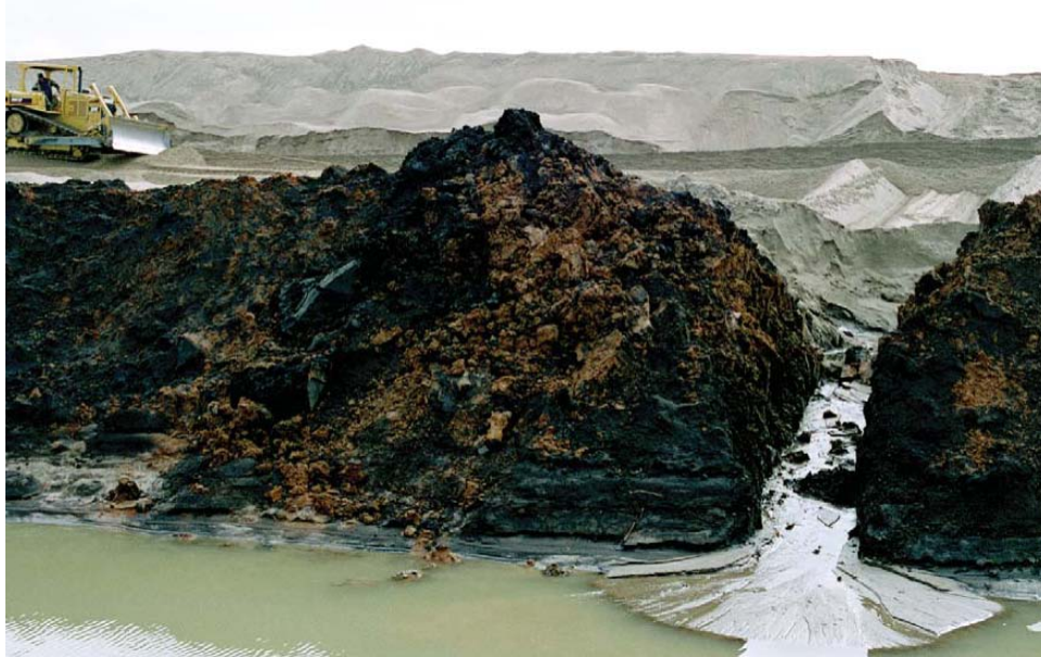
Figure 17. Opening in the containment dike designed to allow runoff of excess water without erosion of the fill material (shown in background). (courtesy of Great Lakes Dredge and Dock Company).
