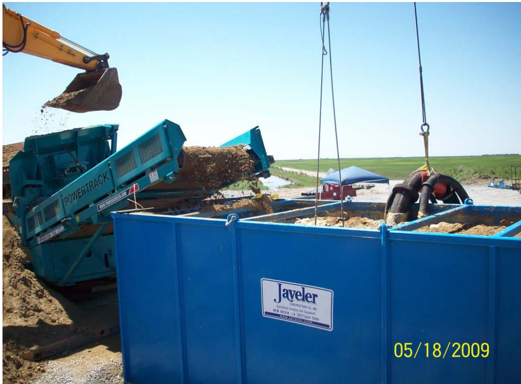
Figure 48. Submersible pump immersed in a transfer hopper that's being loaded with sediment via a conveyor belt operating with water jets (source: Javeler Construction).
