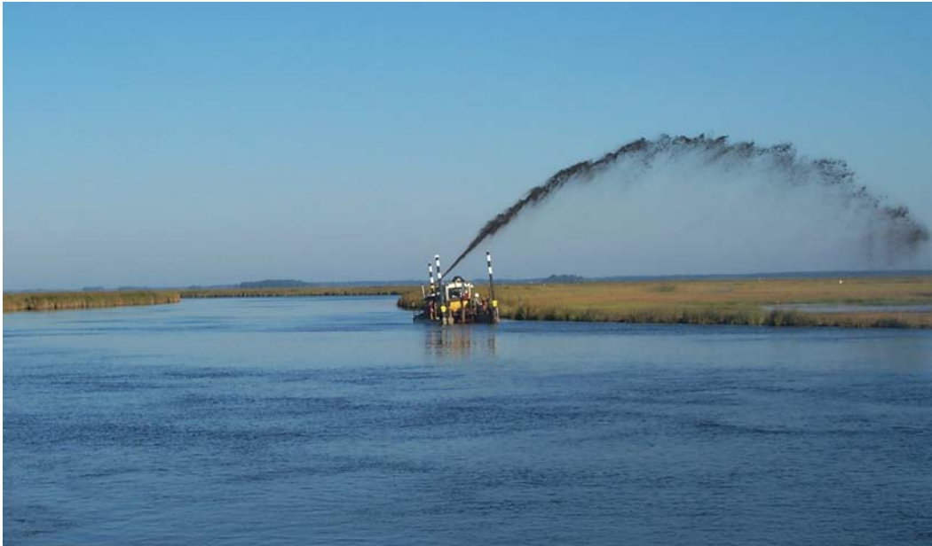
Figure 37. Spray disposal of dredged material (photograph courtesy of Bob Blama, USACE Baltimore District).
