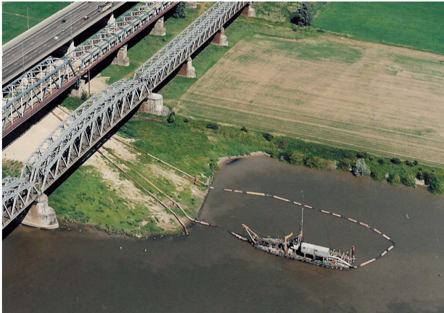
Figure 22. Booster station “Maasvlakte”(source: TU Delft).
