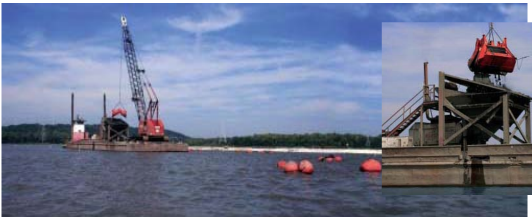
Figure 32. Peoria Riverfront Development, Illinois Upper Mid-sized Island Critical Restoration Project using mechanical bucket dredge and positive displacement (concrete) pump to transport high solids slurry for placement into geotextile containers (photograph courtesy of Cable Arm, Inc.).
