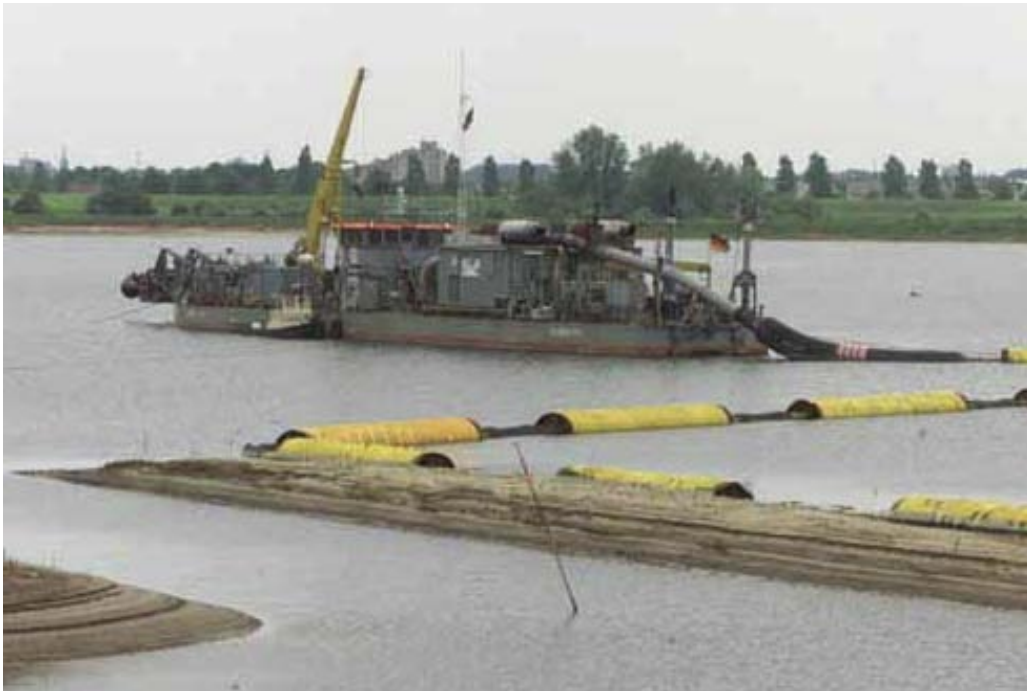
Figure 20. Dredge Nordland at River Maas borrow area (source TU Delft).
