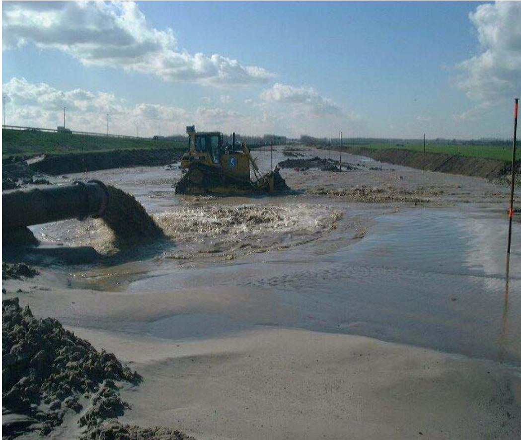
Figure 25. Pipeline discharge at dredged material placement area (source: TU Delft).
