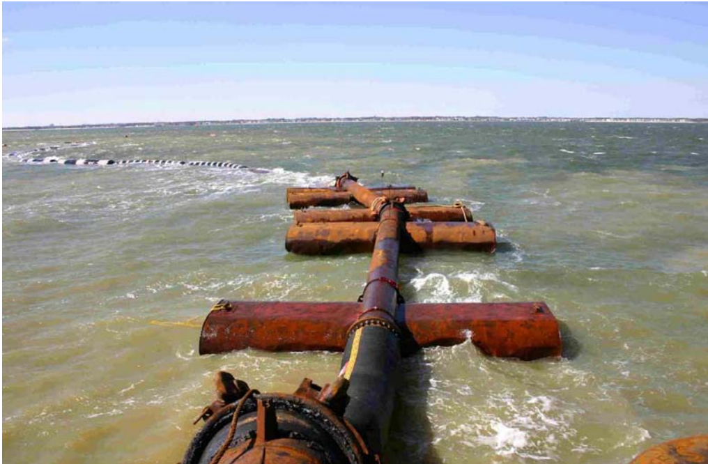
Figure 5. Floating line constructed of steel (see forefront) and rubber-based (see background) material.
