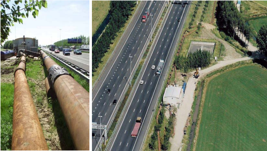
Figure 23. Booster Station “Duinjager” (source: TU Delft).
