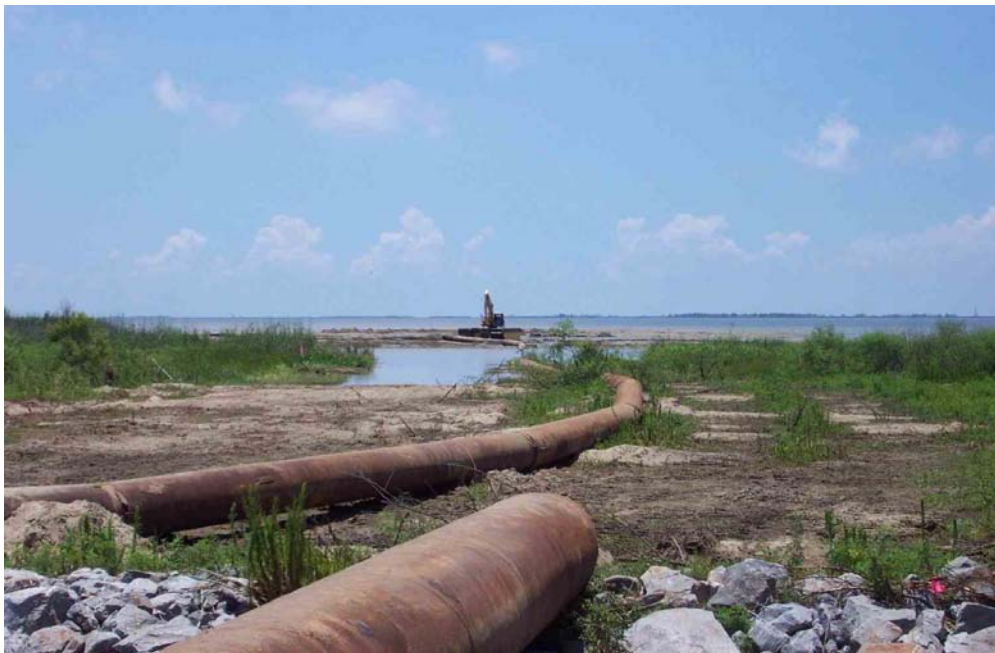
Figure 6. Shore line constructed of steel.
