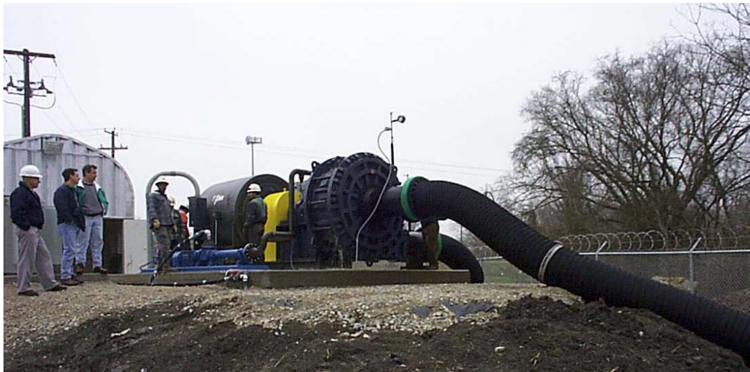
Figure29. Booster pump with AC constant speed motor (source GIW).
