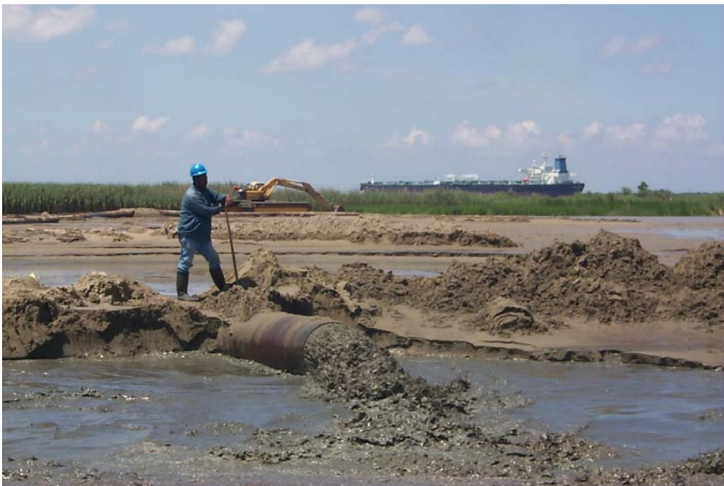
Figure 36. Traditional hydraulic pipeline placement.
