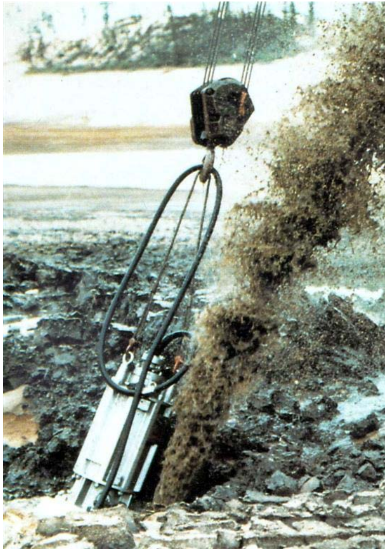
Figure 47. Submersible pump operating without discharge hose connected (source: Javeler Construction).
