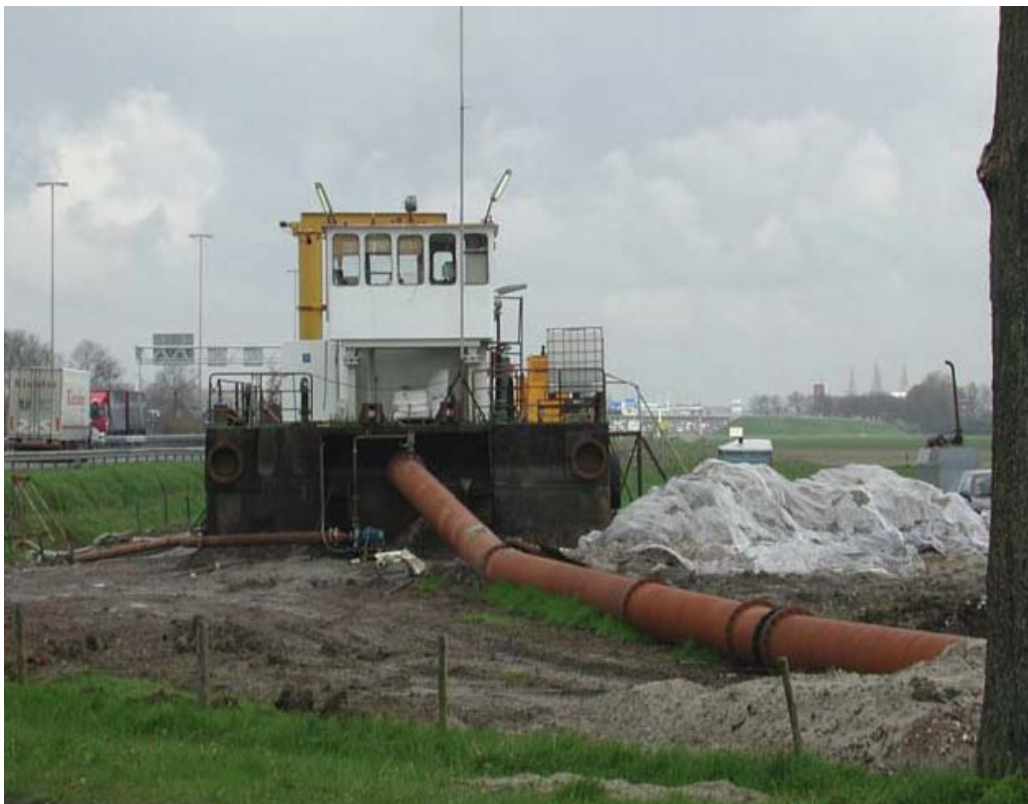
Figure 21. Barge booster station "Bever" (source: TU Delft).
