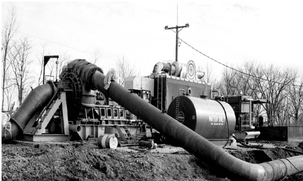
Figure 16. One of two booster pumps used in the I-370 Highway Fill Project (courtesy of Great Lakes Dredge and Dock Company).
