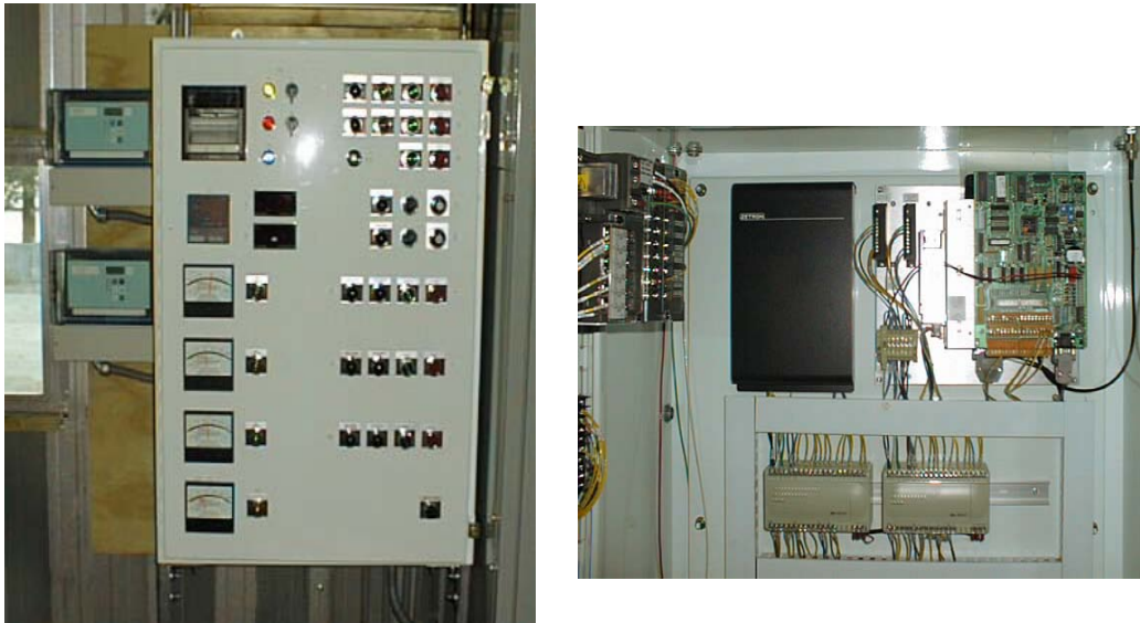
Figure 31. Main control, radio link to dredge, phone line link to remote booster (source: GIW).
