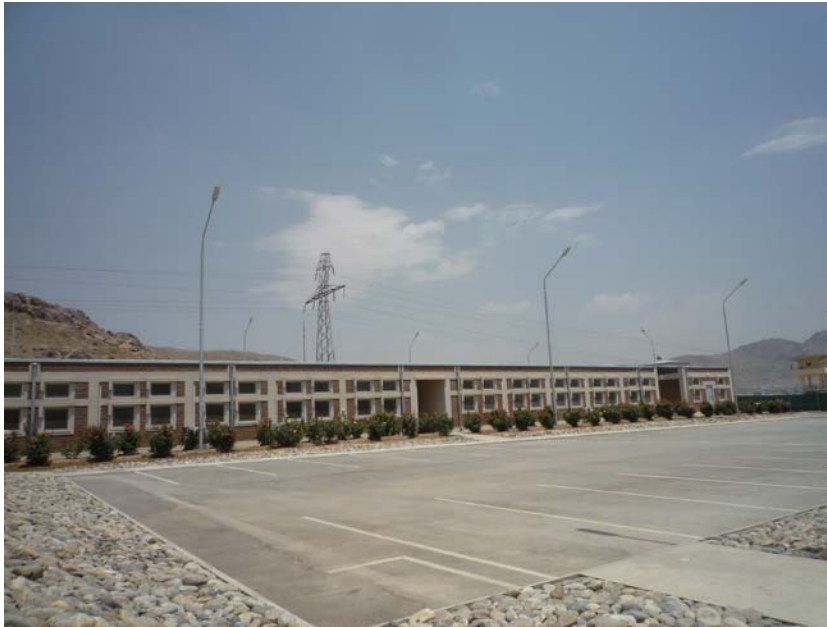
Photograph showing the proximity of the Counter-Narcotics Justice Center to Kabul city power lines. (Source: SIGAR)
