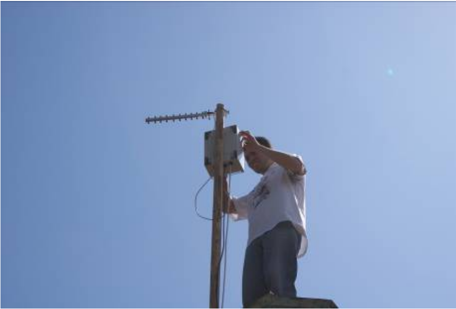
Figure 3 CRD Postdoc Artur Reymers establishing Internet connection of the geomagnetic laboratory to CRD headquarters. Each minute measurement of the 3 components of geomagnetic field will be send to CRD servers for multivariate analysis and alert services.
