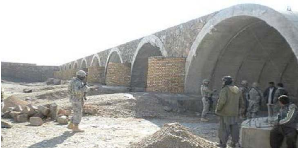
Photo 4: Tojg Bridge Construction, as of January 2010
