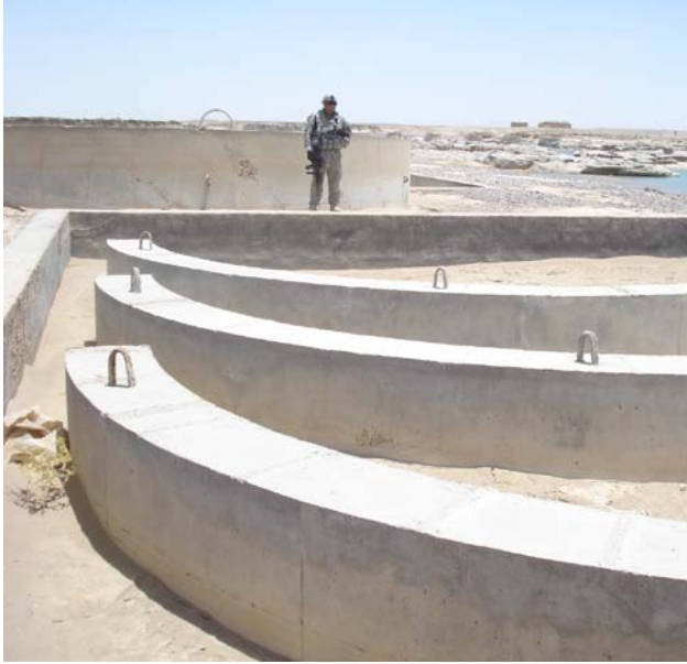
Photo 3: Concrete Arches in a Fabrication Pit
