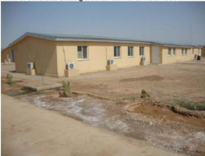
Photo 1: Disturbed Grading around Facilities at Farah ANA Garrison
