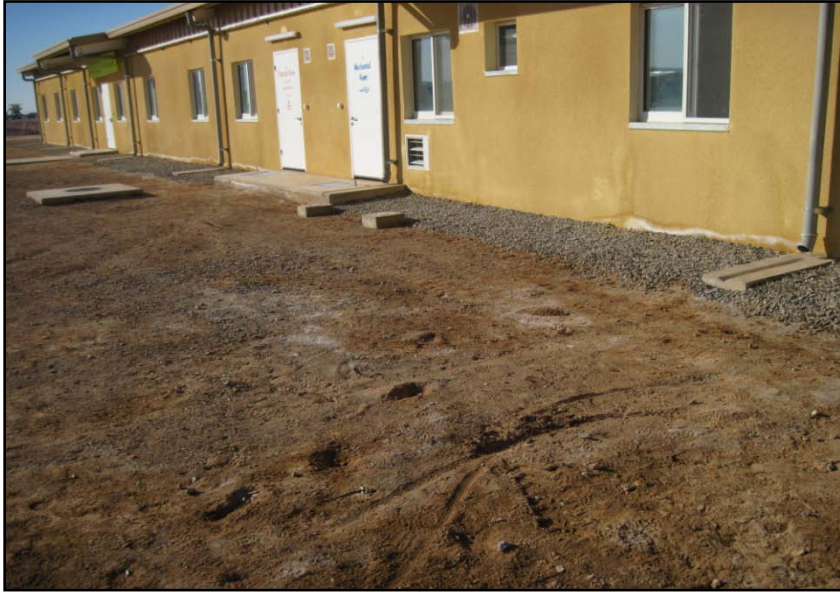
Photo 4: Incomplete Grading around Facilities at Farah ANA Garrison
