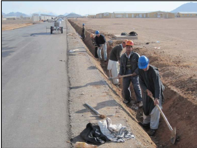
Photo 6: Unlined Ditches at Farah ANA Garrison
