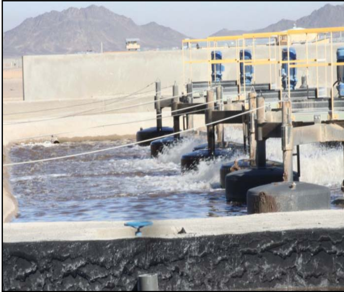
Photo 3: Wastewater Treatment Plant at Farah ANA Garrison
