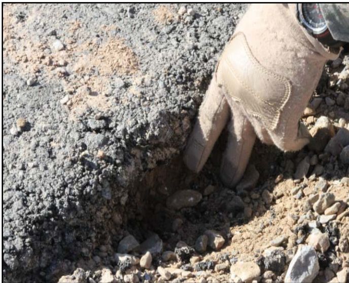
Photo 5: Improperly Compacted Asphalt Paving at Farah ANA Garrison
