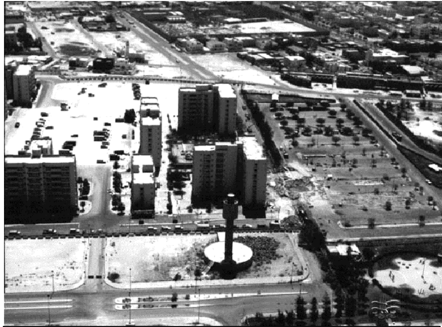
Figure 3-4. Below , Photograph of Khobar Towers After the Bombing ( Source: Report to the President and Congress on Protection of U.S. Forces Deployed Abroad (1996). )
