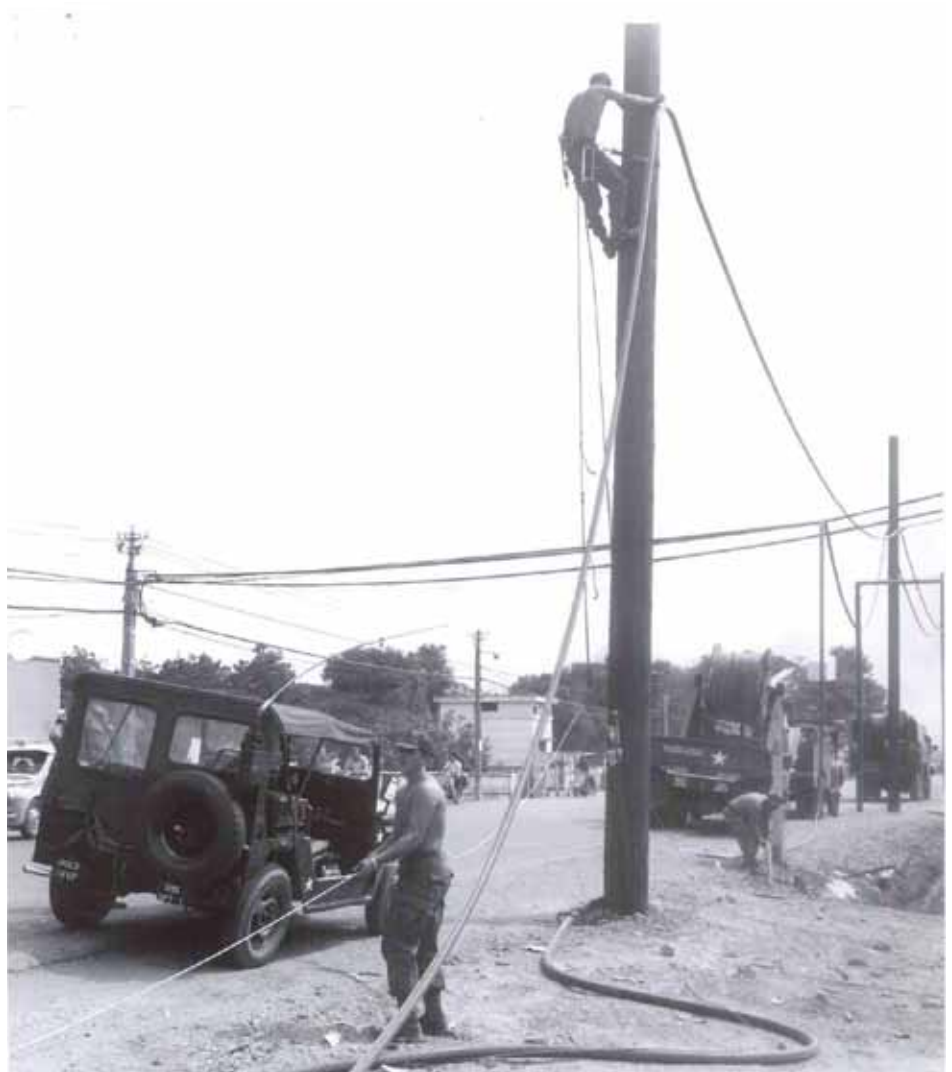
Cable dawgs of U.S. Army STRATCOM's 69th Signal Battalion effect communications cable repairs following a fire fight on Plantation Road in Saigon, South Vietnam in April 1969
