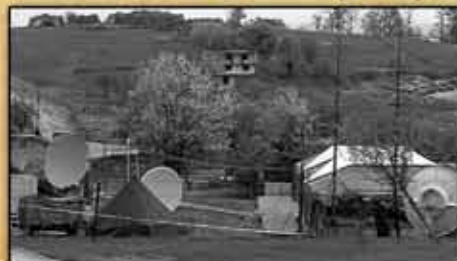
Communications site - Bosnia-Herzegovina, early 1990s
