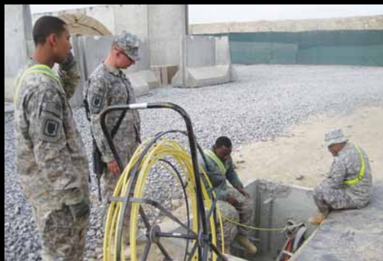
Members of the 57th Expeditionary Signal Battalion lay fiber optic cable at U.S. Air Force Camp Davis January 2010 to provide connectivity to the aviation brigade at Kandahar Airfield.
