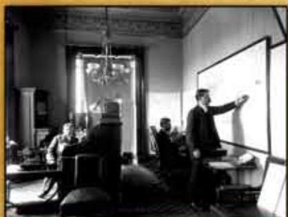
White House Communications Room, 1898
