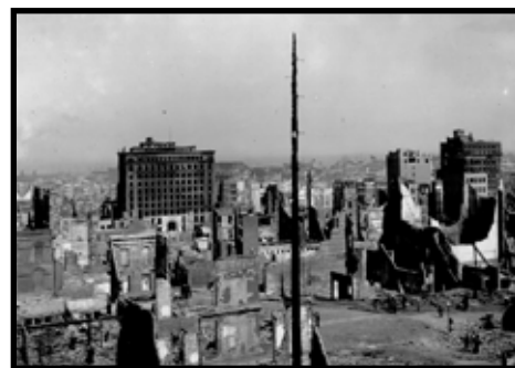
San Francisco earthquake, 1906
