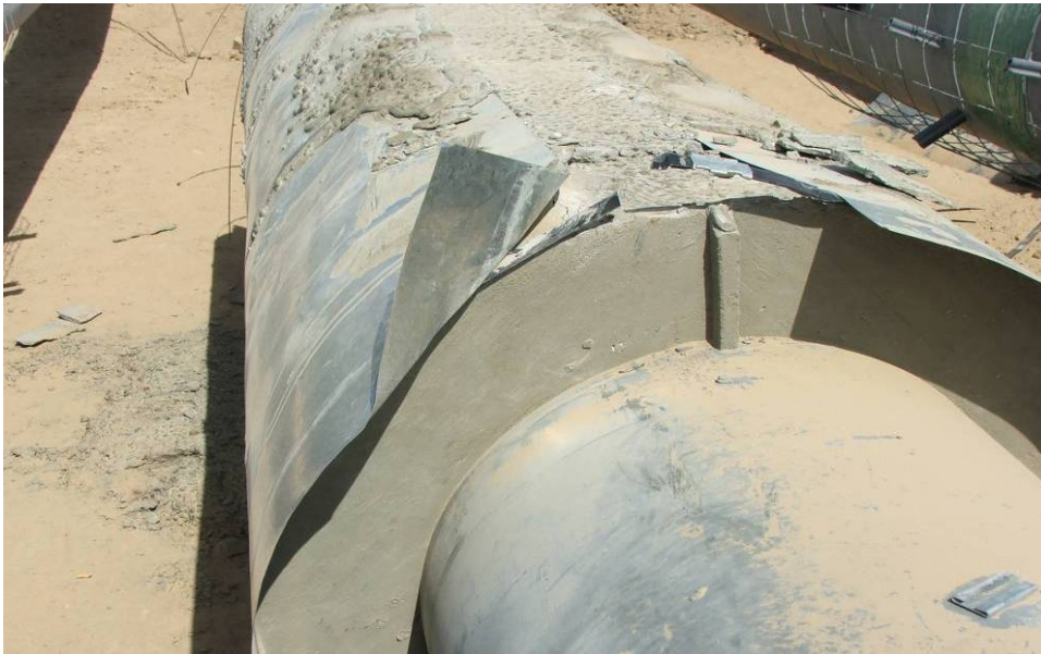
Site Photo 7: Section of Pipe Encased In Concrete
