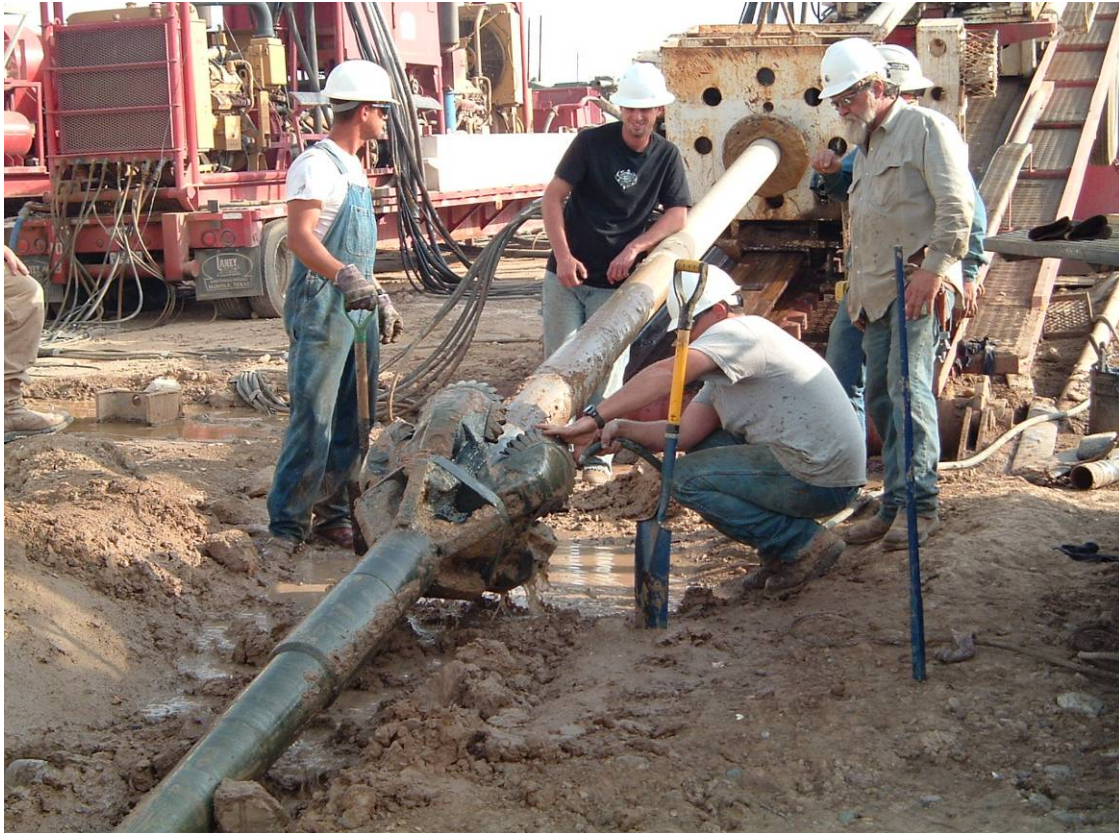
Site Picture 3: HDD Rig with Backreamer
