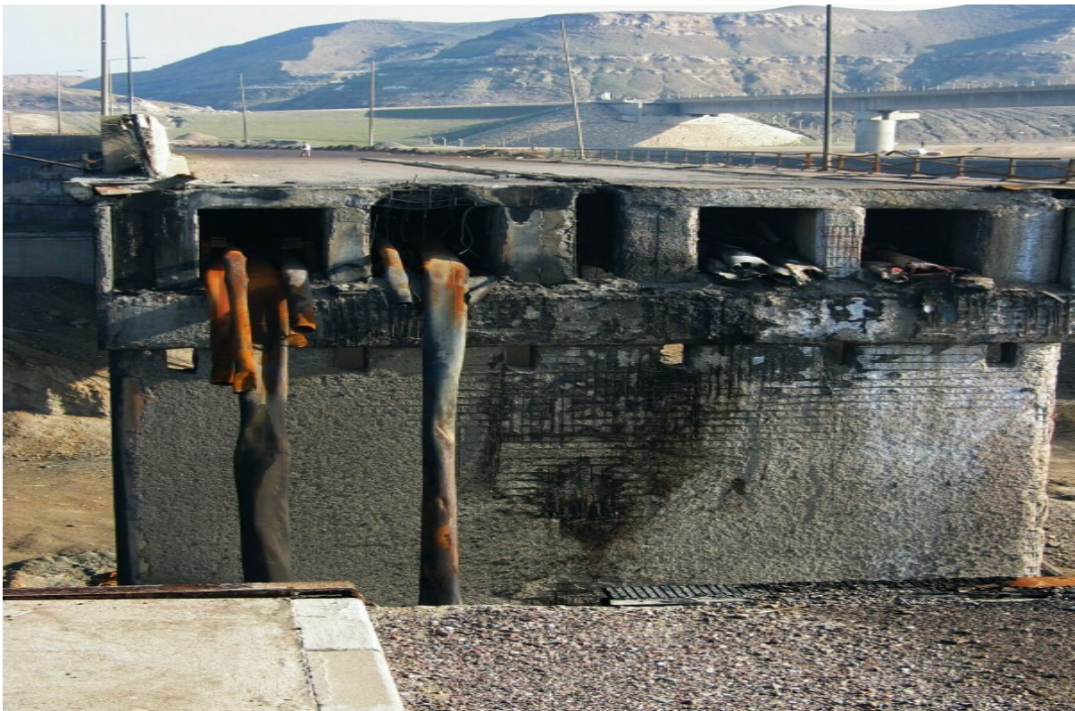
Site Photo 2: Bridge cross section showing the melted pipes from the bomb damage
