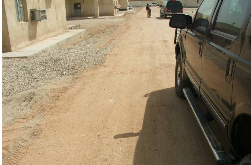
Site Photo 16. Compacted subbase material for one of the new roads under construction
