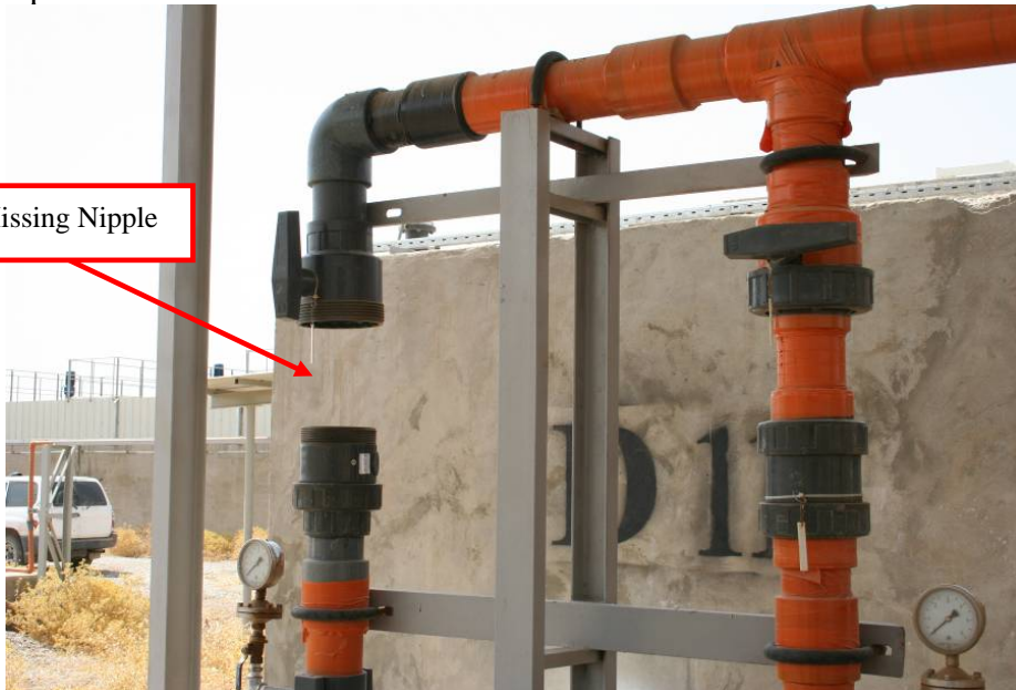
Site Photo 22. Missing nipple meant that back flushing could not be performed.
