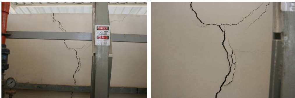
Site Photos 11 and 12. Vertical cracks were present in the inner rear wall of the pump station.
