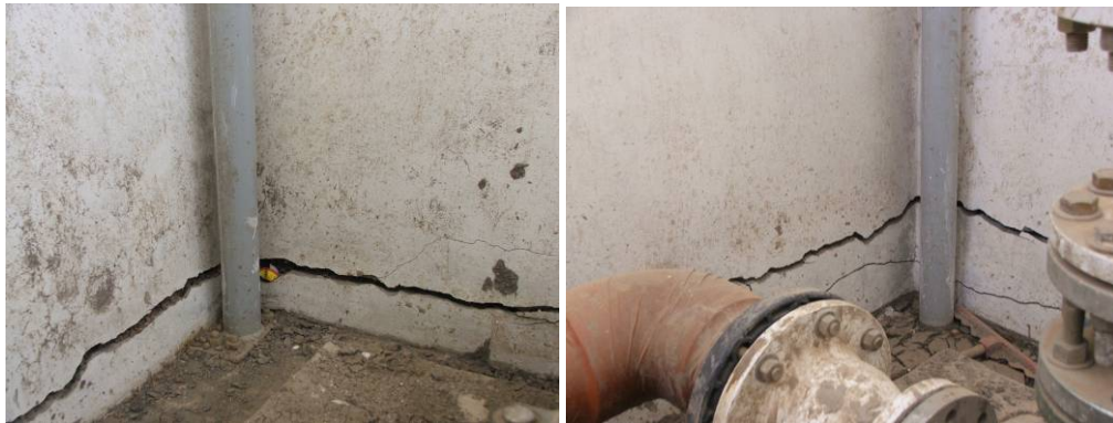
Site Photos 15 and 16. Horizontal cracks near the floor at opposite corners of the G-03 building.
