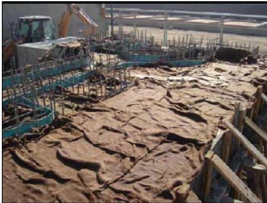
QA Photo 8. Concrete covered with burlap to prevent too rapid drying and decreased strength (from QA Report 3 Oct 2005).
