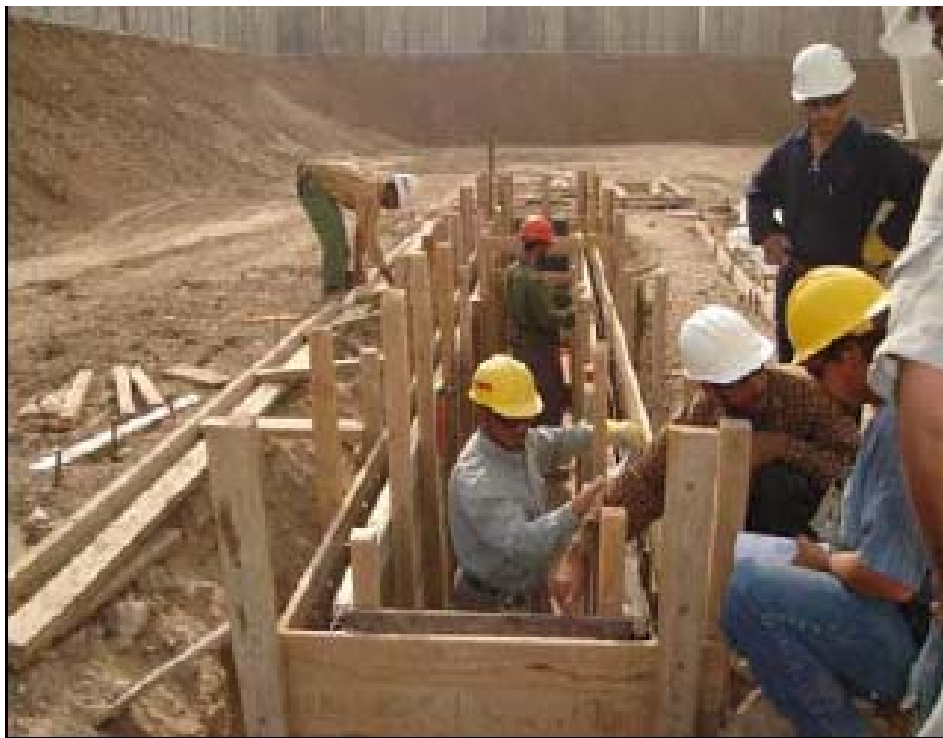
QA Photo 6. Good form techniques were used to build a sub-grade foundation with supervisors on site (from QA Report 11 Oct 2005).
