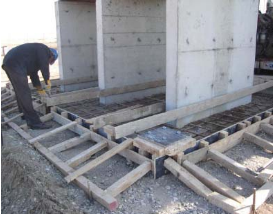
QA Photo 5. Flatwork form with clear / sufficiently sized lumber and proper brace placement (from QA Report 14 Dec 2005).
