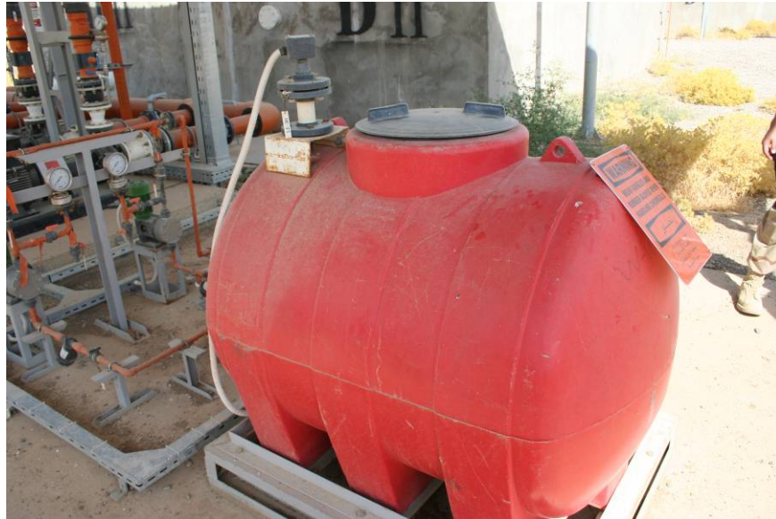
Site Photos 19. Chlorination system included a holding tank for Sodium Hypochlorite (NaOCL).
