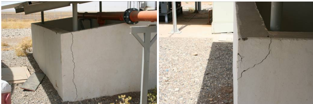
Site Photos 17 and 18. Vertical cracks wound their way to the outer corners of the rear wall.
