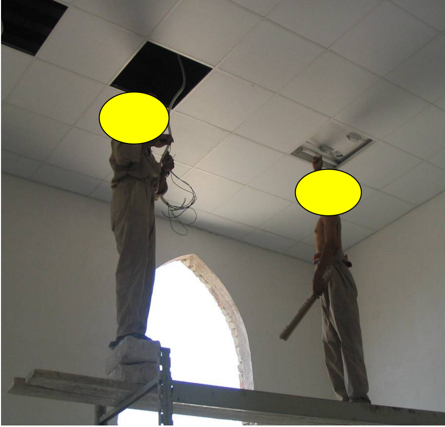
Site Photos 3 and 4. Installation of electrical wiring in the MOD HQ building (Photos courtesy of Laguna Construction)
