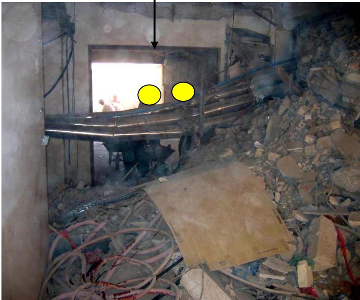
Site Photos 1 and 2. Interior and exterior JDAM bomb damage to the MOD HQ building (Photos courtesy of Laguna Construction)
