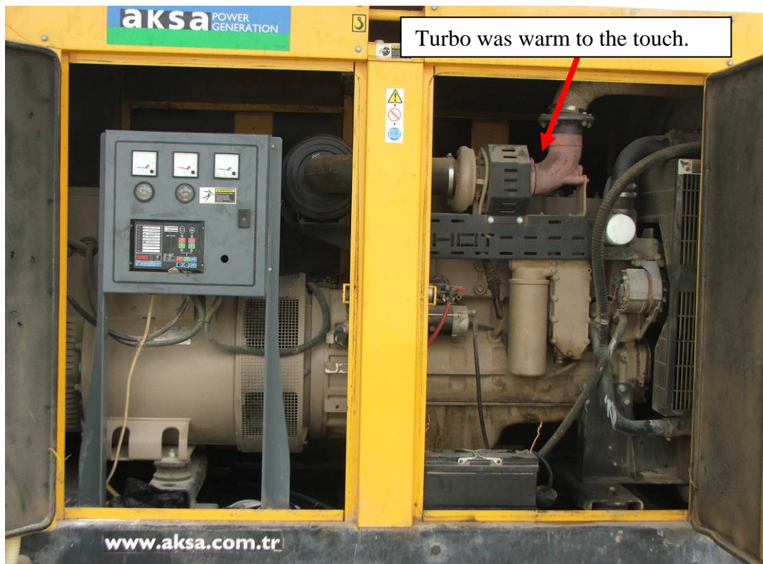
Site Photo 1. The generator installed per requirements appeared completely operational without any signs of neglect. When checked, the oil level was full and did not feel gritty. Belts and hoses appeared serviceable.
