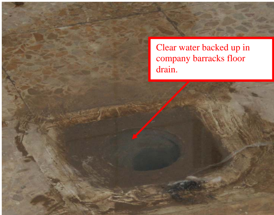
Site Photo 6. Clear water backed up in floor drain of company barracks.
