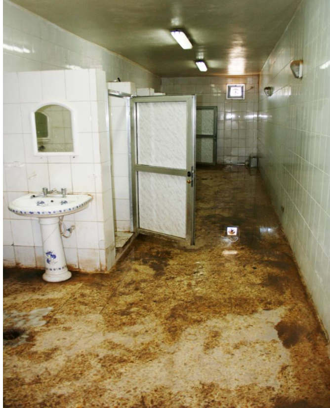
Site Photo 5. Drainage problem in barracks bathroom.
