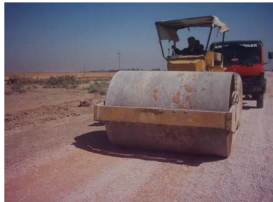
Site Photo 4. Compacting the sub-base with a steel wheeled roller – Photo provided by USACE
