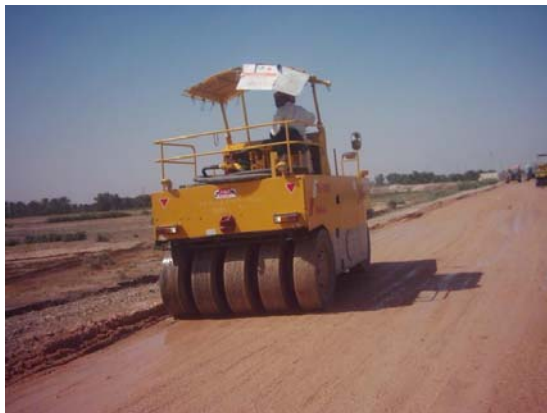
Site Photo 3. Compacting the sub-base with a pneumatic rubber tired roller – Photo provided by USACE
