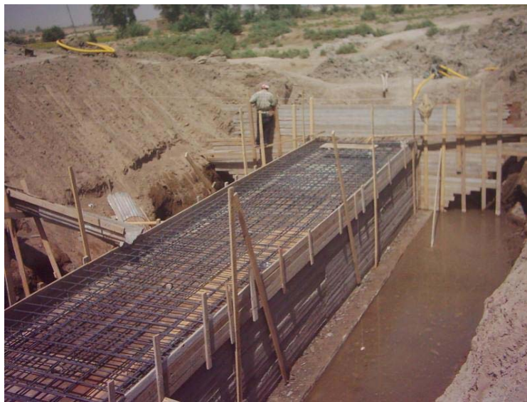
Site Photo 11. Construction of reinforced concrete box culvert – Photo provided by USACE.
