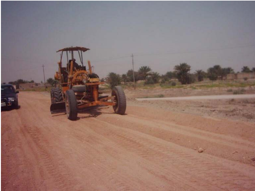
Site Photo 1. Contractor motor grader leveling the sub-base – Photo provided by USACE
