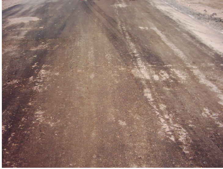
Site Photo 7. Lack of sufficient prime coat on sub-base prior to paving – Photo provided by USACE
