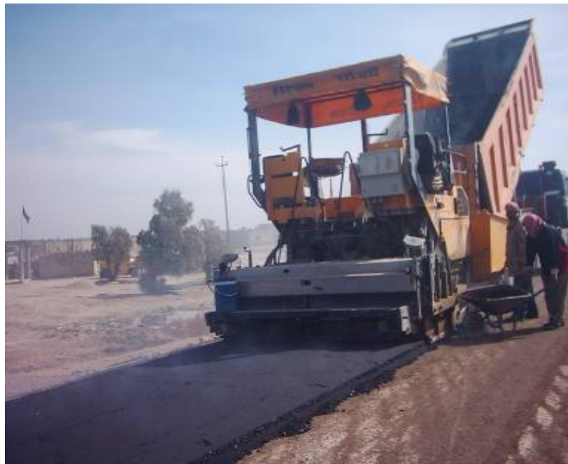
Site Photo 5. Placing and spreading asphalt concrete pavement –Photo provided by USACE
