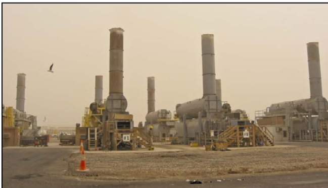
Figure 4. Incinerators in operation at Joint Base Balad, Iraq, November 2009. (Photo provided by the author.)
