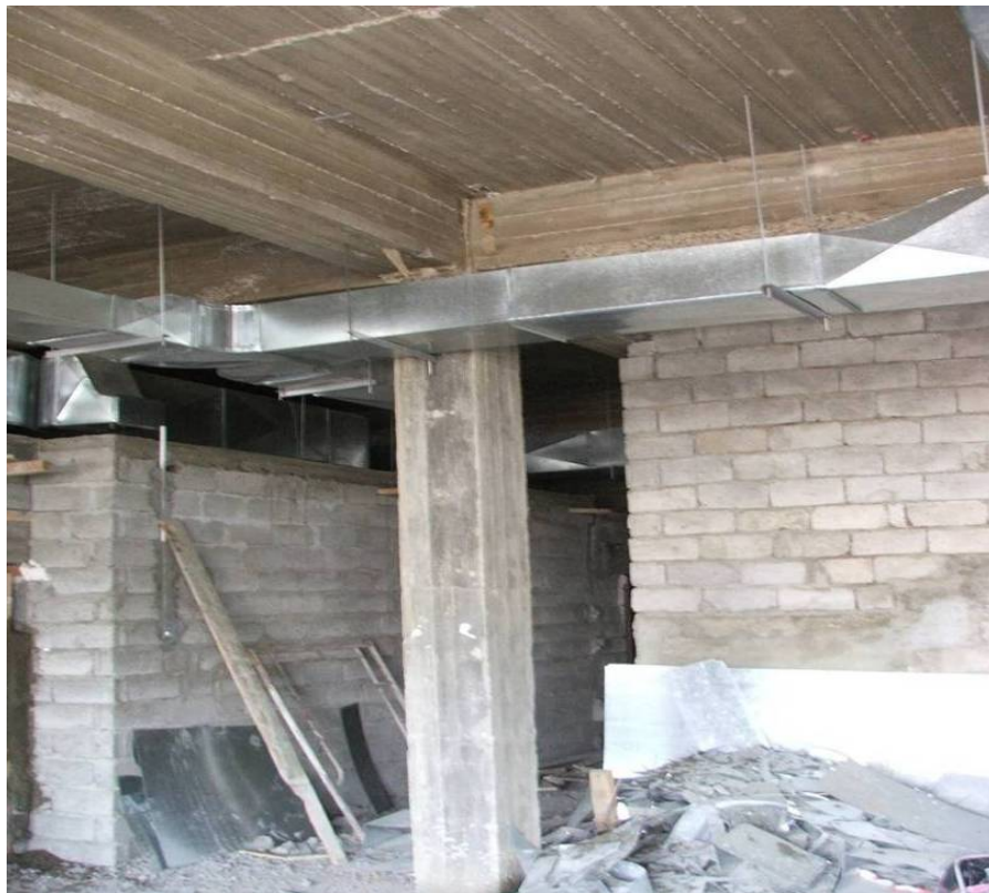
Site Photo 4. Column that is not plumb (PHC Hai Alasra Wa Al Mafqoodeen)
