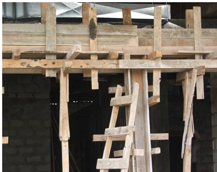
Site Photo 78. Example of remaining formwork
