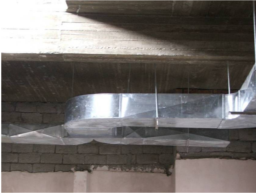
Site Photo 35. Installation of ventilation ductwork
