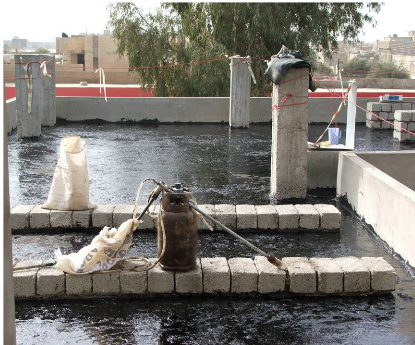
Site Photo 43. Tar applied to the roof
