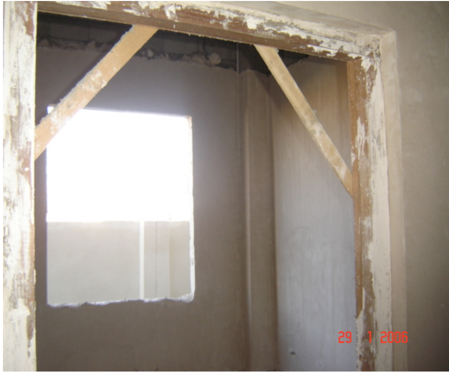
Site Photo 74. Example of window without window frame and grilles (Photo courtesy of the USACE)
