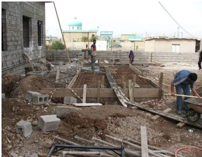
Site Photo 76. Rebar and formwork for the top of the septic tank
