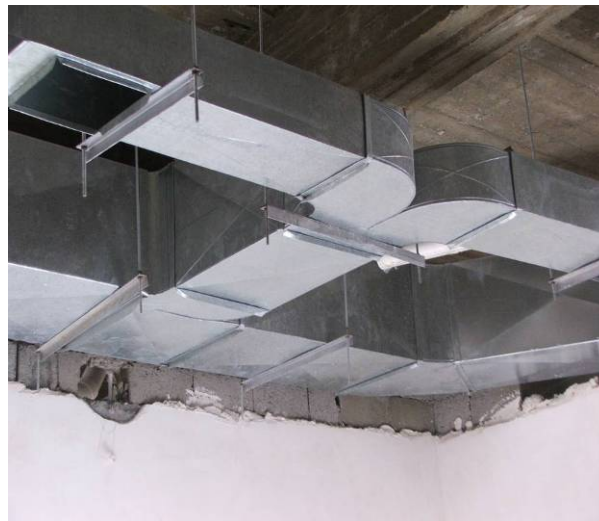
Site Photo 45. Ventilation ductwork
