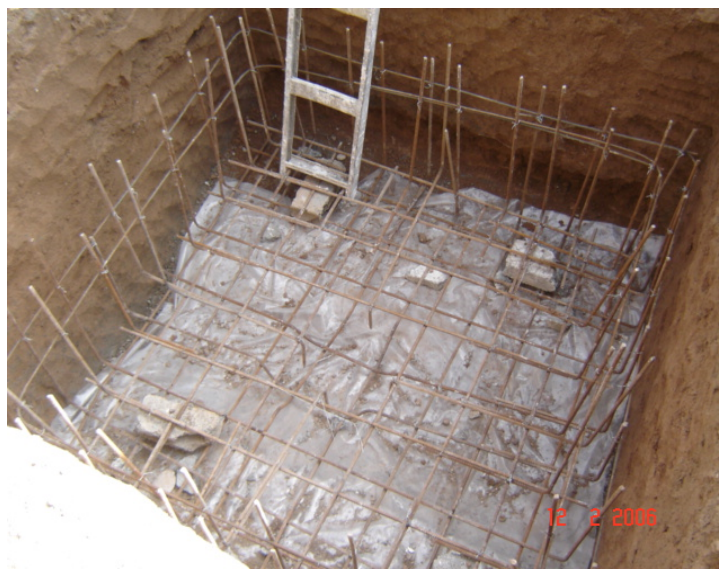
Site Photo 63. Excavated hole for septic tank (Photo courtesy of the USACE)
