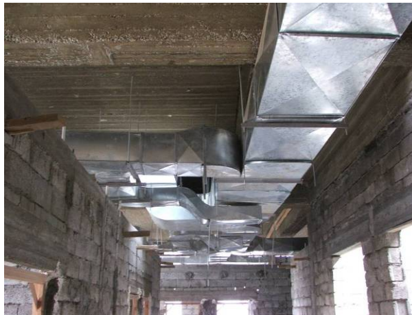
Site Photo 82. Completed ventilation ductwork
