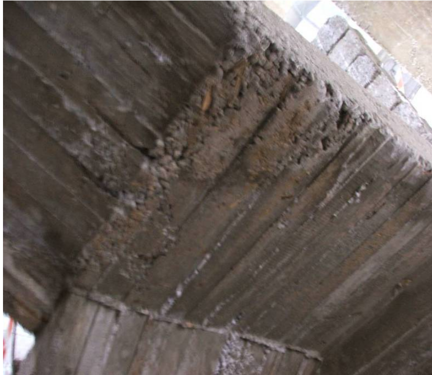
Site Photo 10. Concrete segregation underneath stairwell (PHC Hai Al Wesity)
