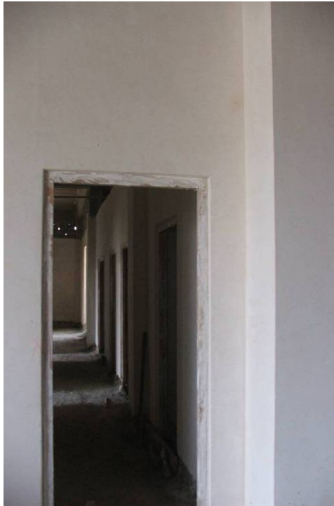
Site Photo 39. Example of completed doorframes
