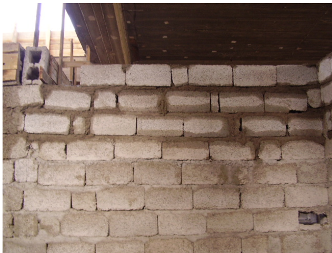
Site Photo 54. Example of different sized blocks in wall construction (Photo courtesy of the USACE)
