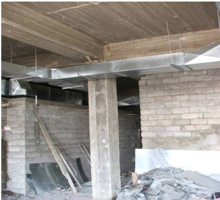
Site Photo 4. Column that is not plumb (PHC Hai Alasra Wa Al Mafqodeen)
