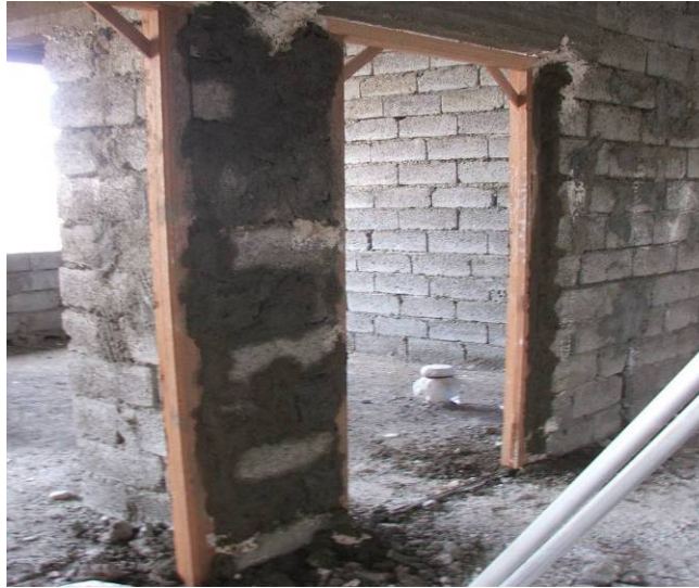
Site Photo 85. Partially installed doorframe
