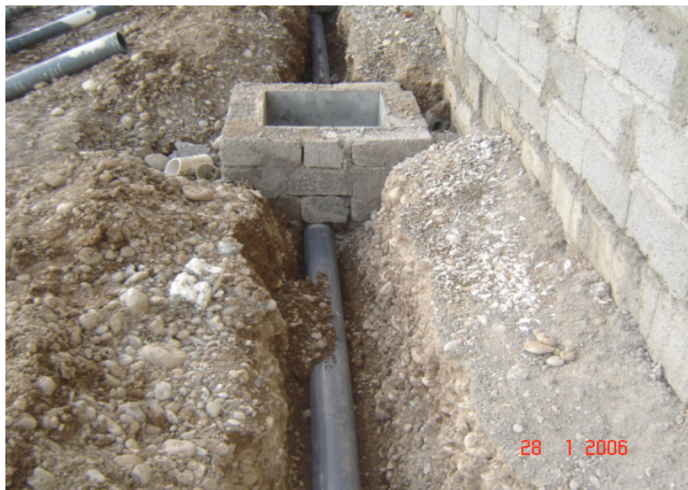
Site Photo 71. Partial installation of sewer drain (Photo courtesy of the USACE)
