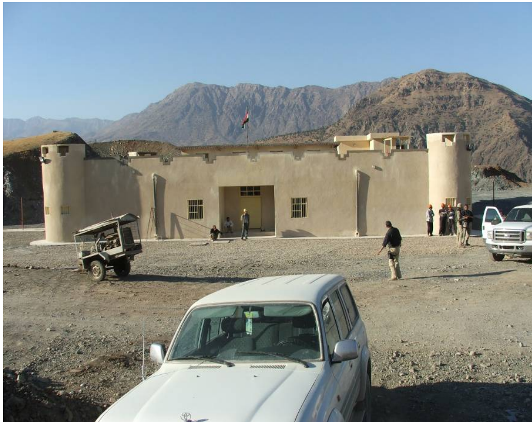
Site Photo 30. Front Exterior View of Border Post (Marwa #628 Border Post)
