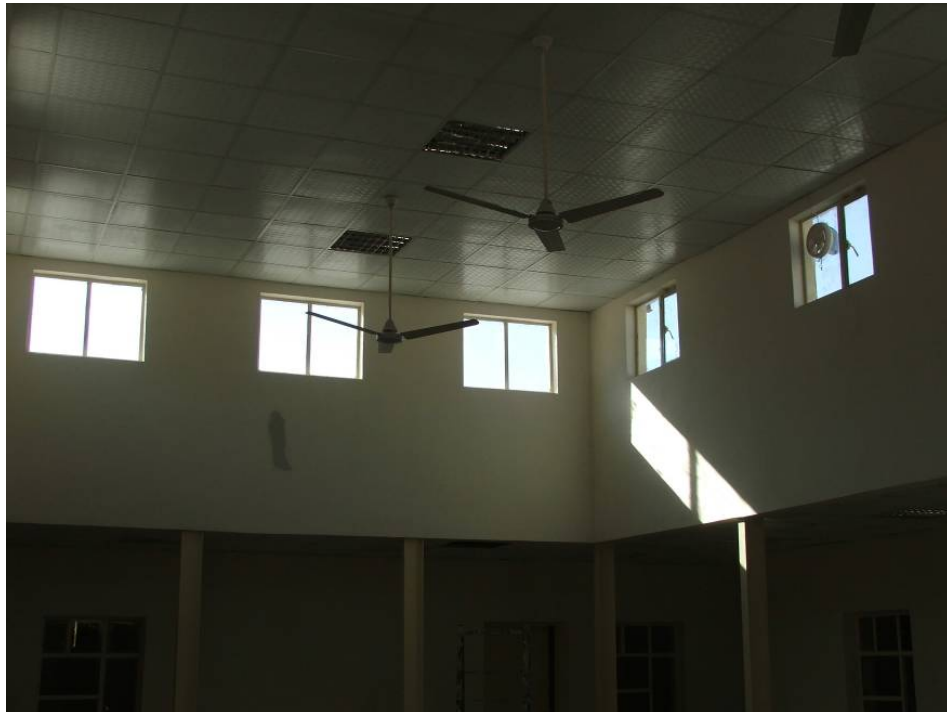
Site Photo 41. Interior Atrium (Azmic #602 Border Post)
