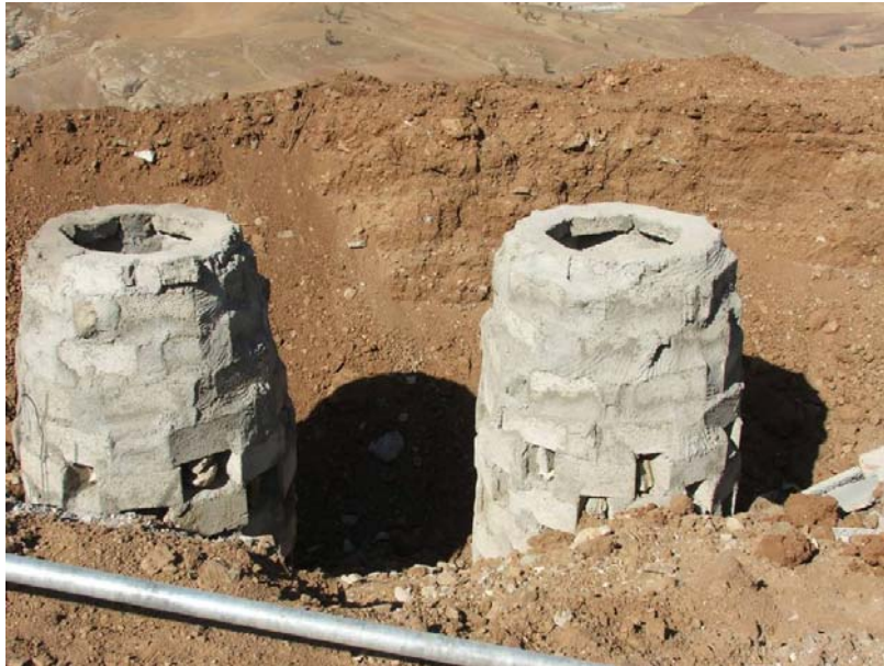
Site Photo 58. Two Soakaways (Issawa #604 Border Post)
