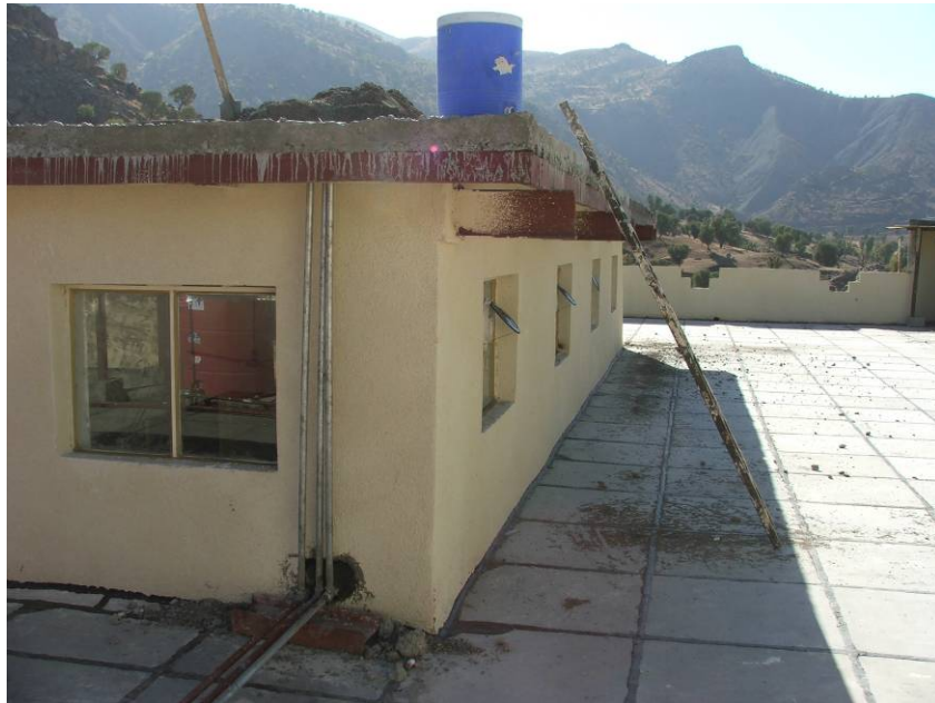
Site Photo 42. External View of Atrium (Azmic #602 Border Post)
