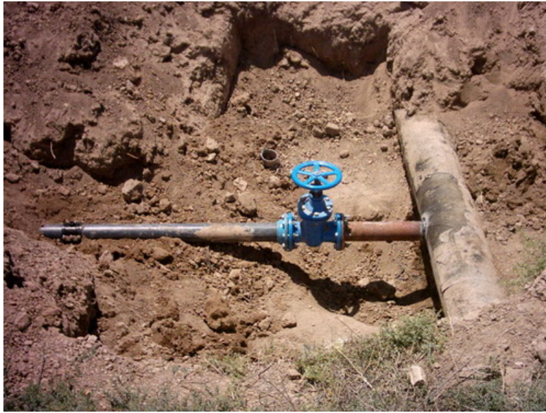
Photo 3: 110 mm connection to 300 mm existing pipe
