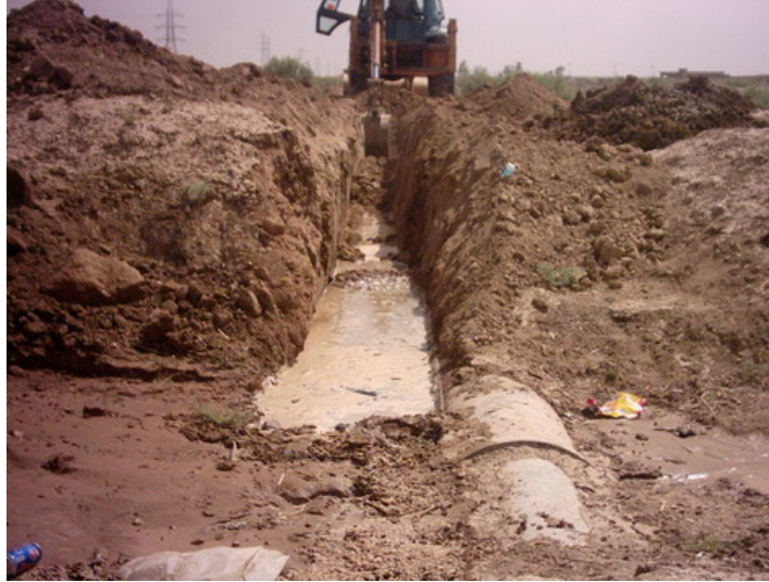
Photo 4: Excavation to locate illegal connections
