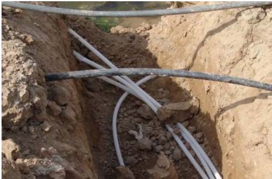
Photo 9: Placement of 15 millimeter water lines in excavation
