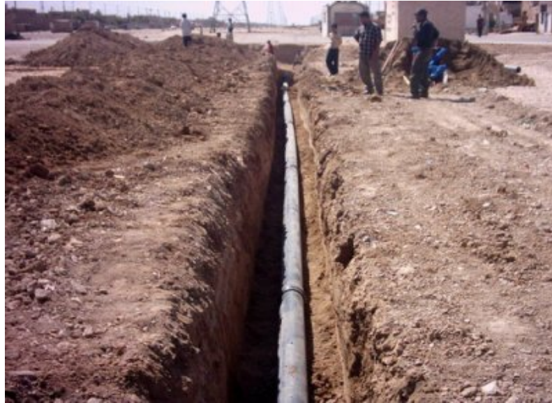
Photo 2: Installation of 200 mm UPVC pipeline
