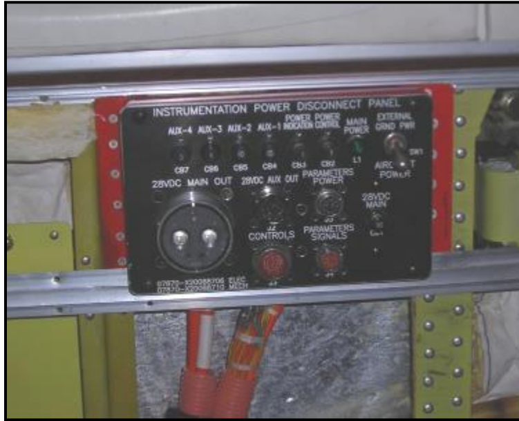
Figure B2. Instrumentation Power Disconnect Panel
