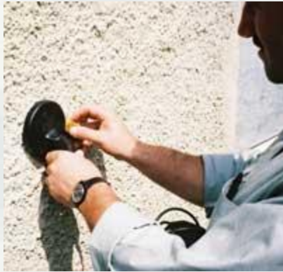
Locate the Metal Ties
