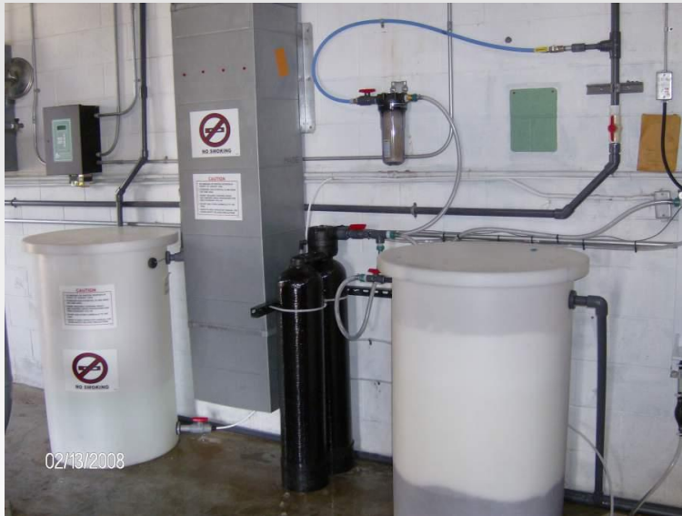
Brine and Oxidant Tanks
