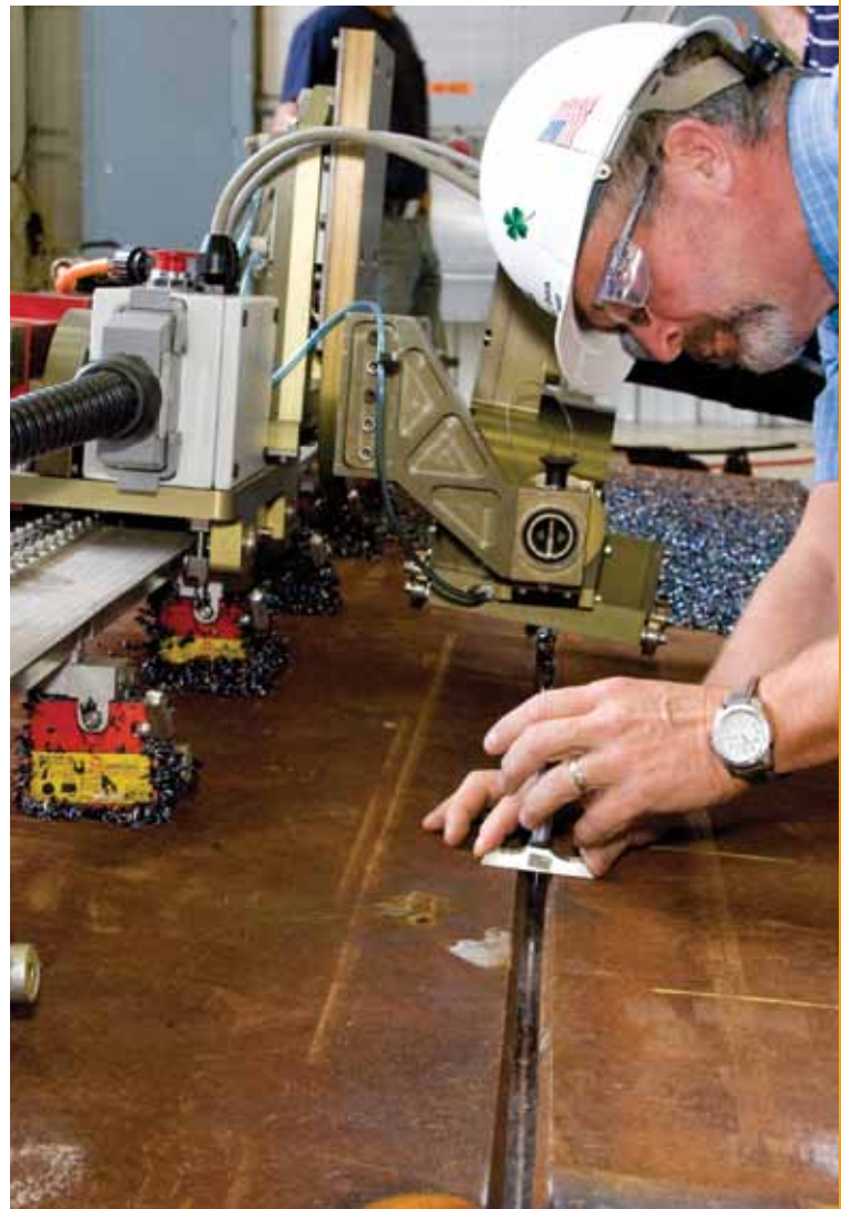
The track weld shaver system shown on the opposite page was modified to perform back gouging on DDG 1000, which will save $400,000 in labor per hull. Bath Iron Works photo
