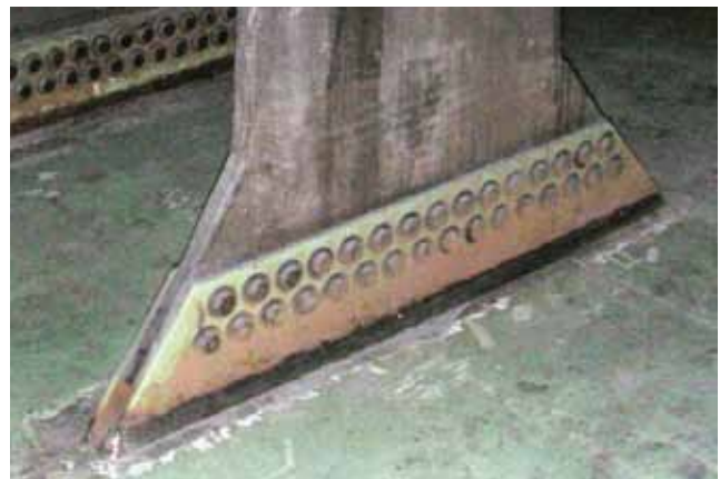
Improved welding and cutting processes to connect the DDG 1000 deckhouse to the deck will save more than $840,000 for the ship class. NGSB-GC photo
