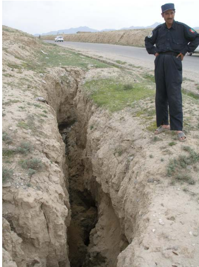
Figure 4. Example of erosion removing the soils near the road.
