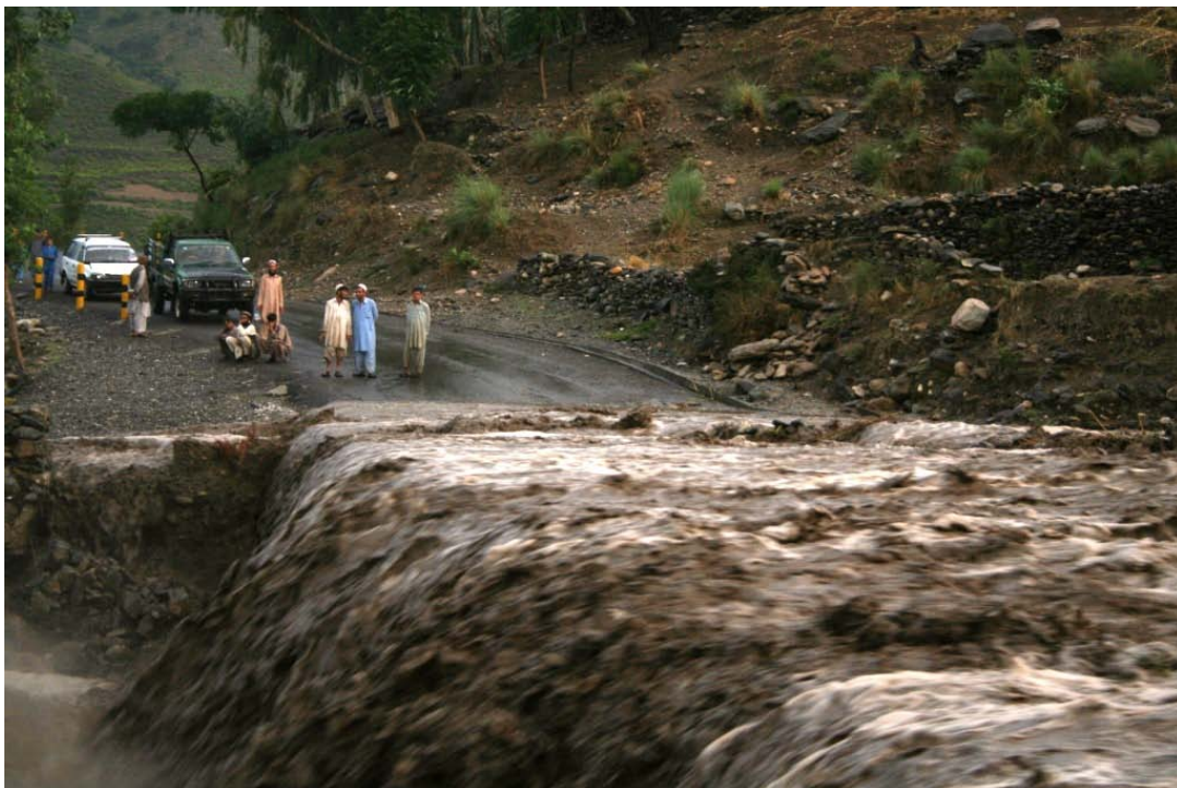
Figure 3. Road washed out during the wet season.
