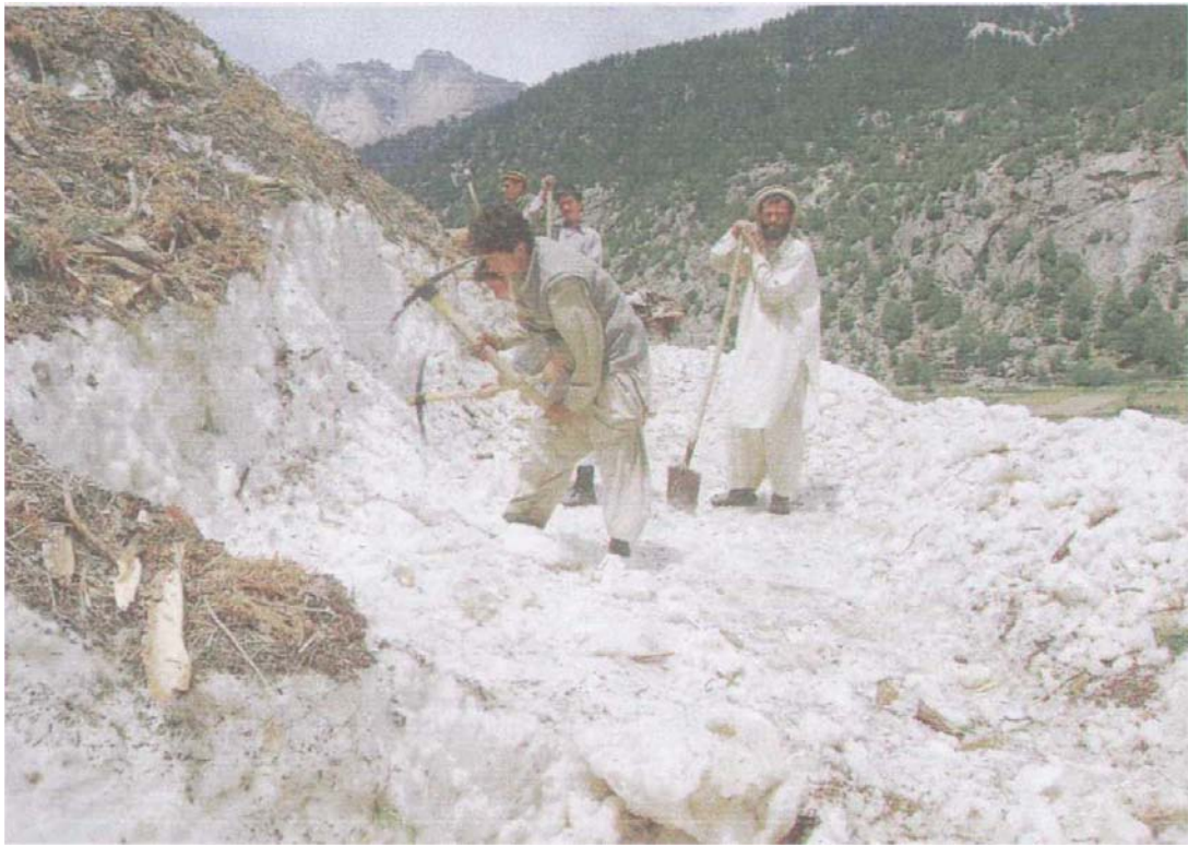
Figure 5. Building a road using manual labor (Afghans).
