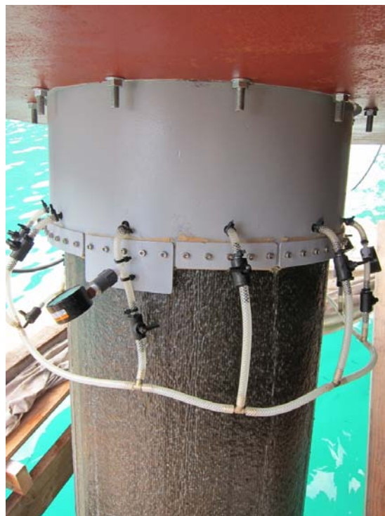
Figure 261. Upper Guide Ring with Water Manifold Attachment
