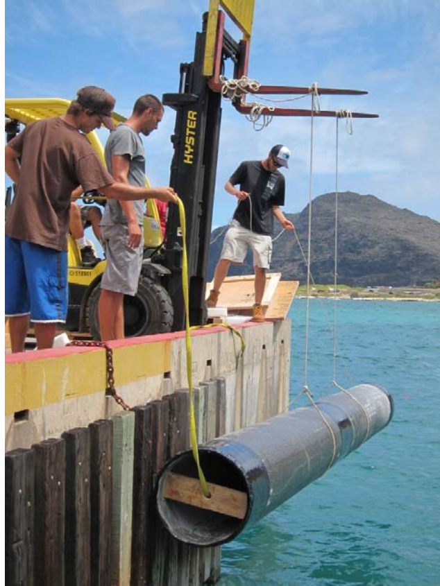
Figure 263. Lowering CWP into the water
