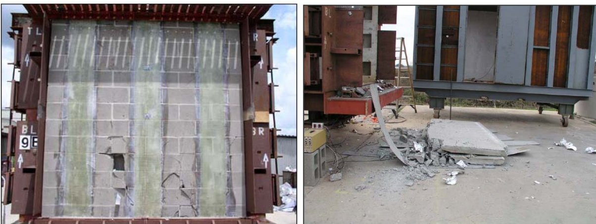
Figure 3. Damage levels of CMU walls upgraded with FRP (BakerRisk, 2004; BakerRisk, 2008)
