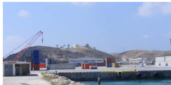
Fig.8 View from Berth 21 to Port Control
