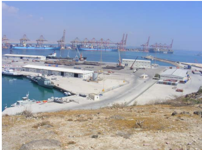
Fig.3 View North to Container Terminal
