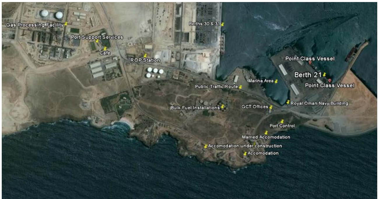
Fig. 5 GCT & EXPOSED SITES TO SOUTH
