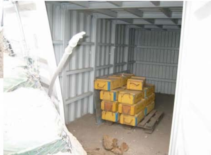
Right container – internal view
