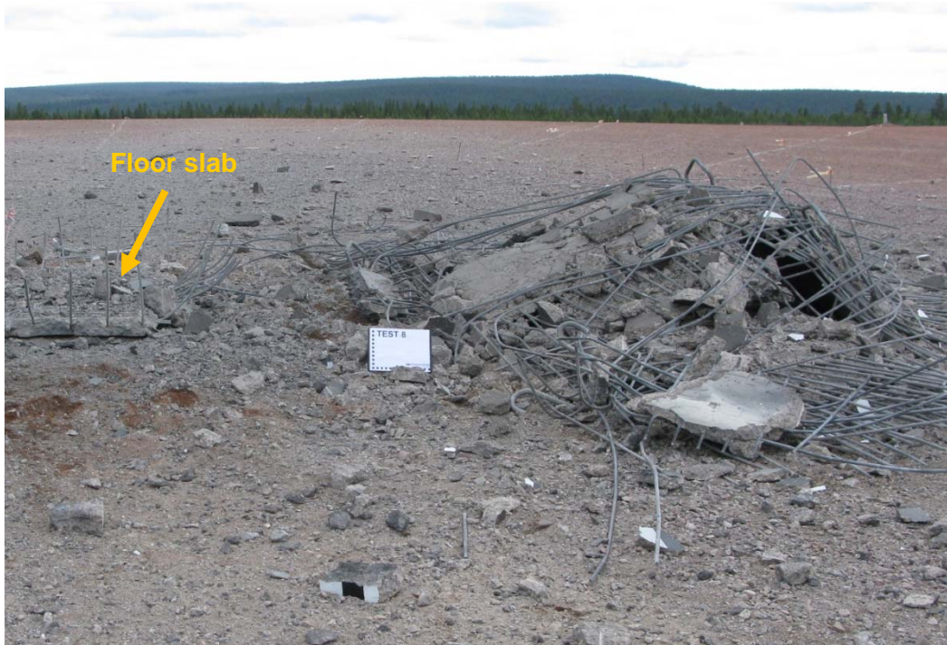
Figure 9. Concrete from the roof and upper section of the walls found next to the floor slab in the one shell test.
