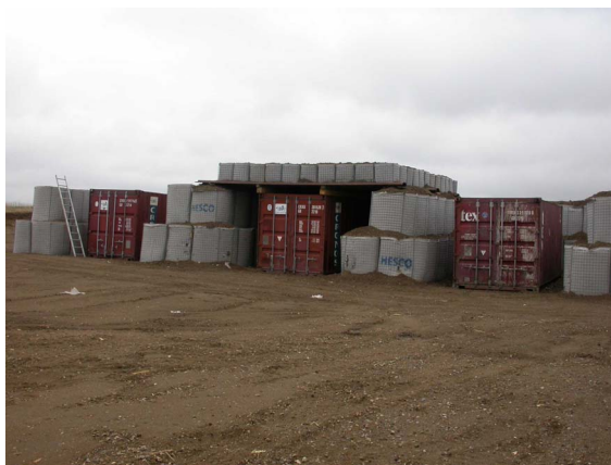
Figure 6. Physical protection of an ES structure with barricades (HESCO) and overhead protection
