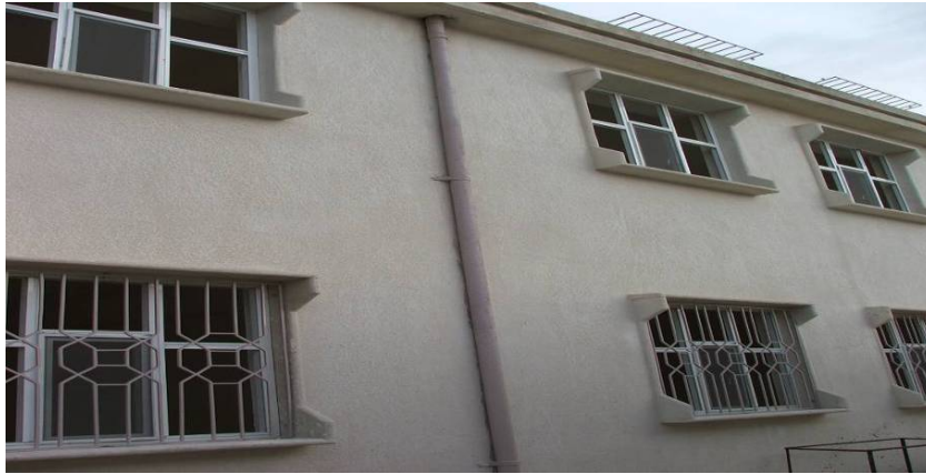
Site Photo 8. Exterior showing painted cement finish and windows
