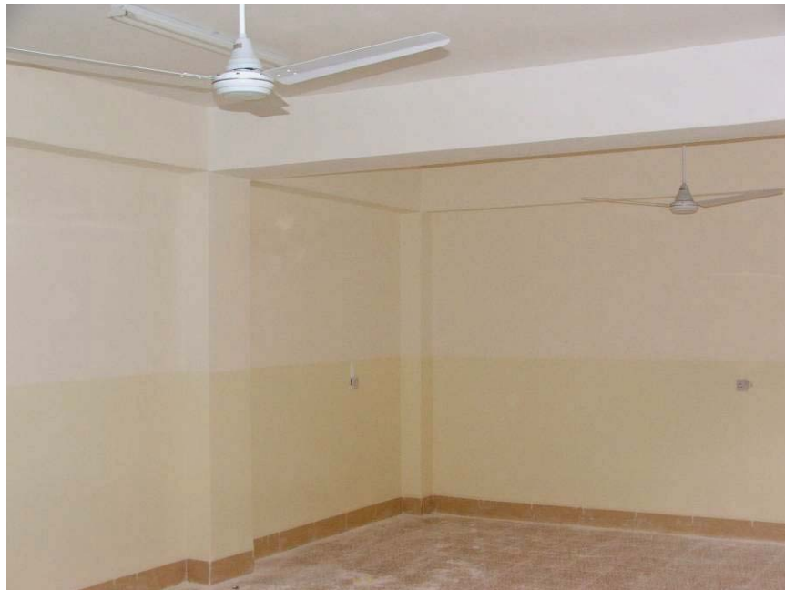
Site Photo 6. Ceiling fan installation
