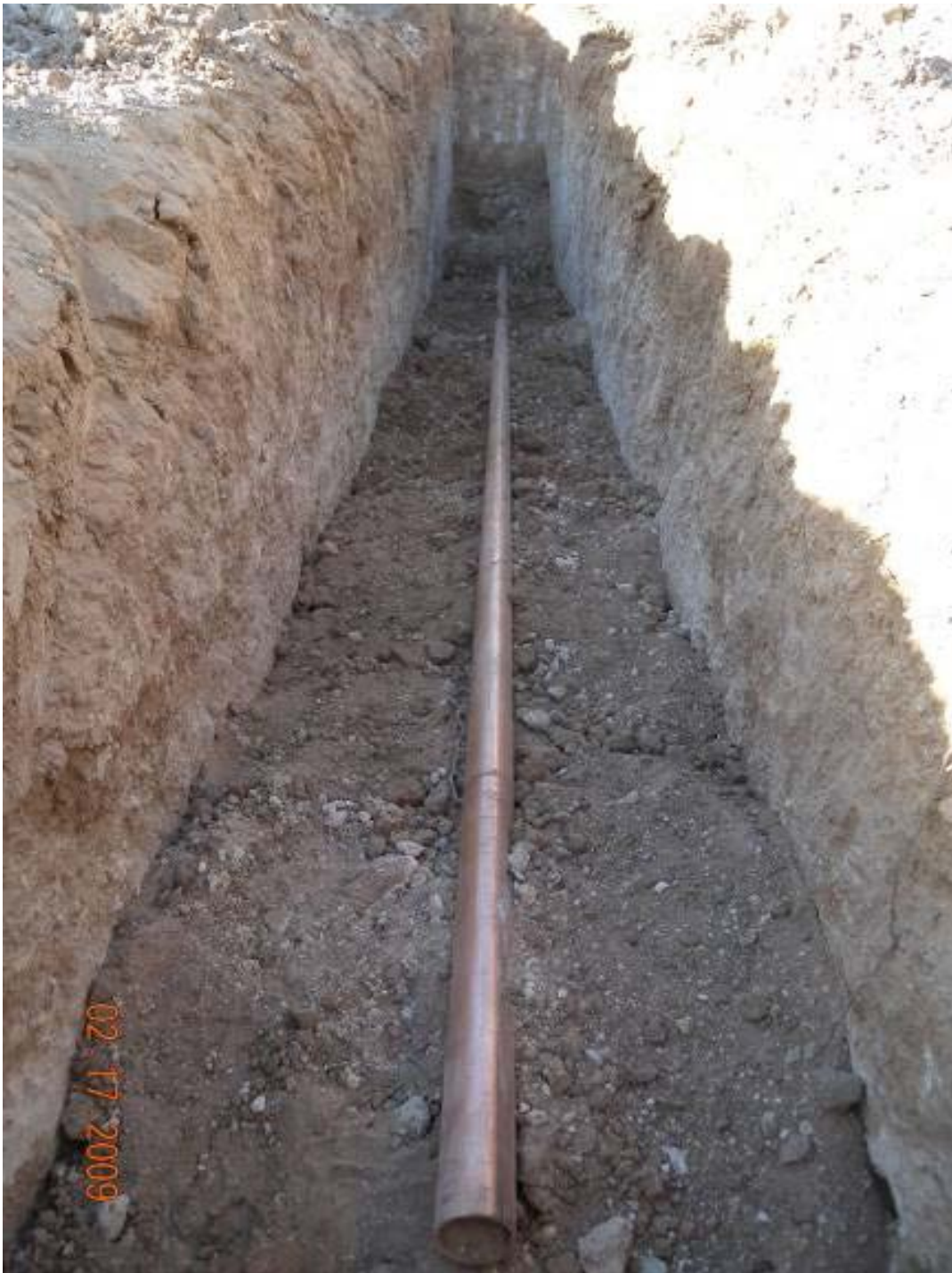
Figure 9. Copper pipe: 2-in. (5 -cm) diameter.
