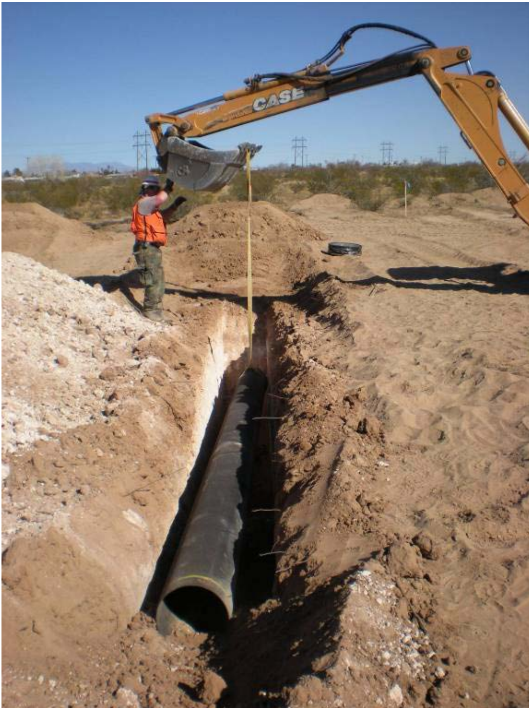
Figure 11. Ductile iron pipe: 12-in. (30.5-cm).
