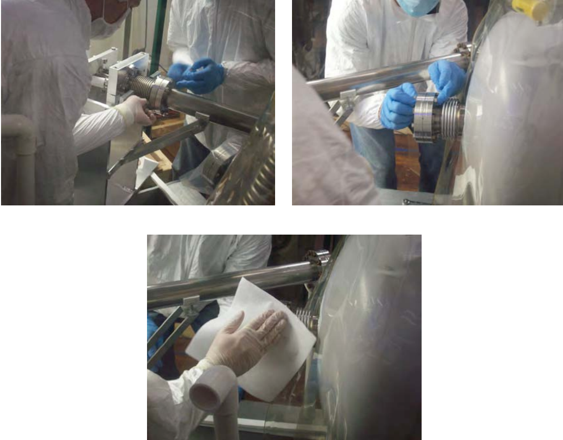
Figure 47. The surrogate beam tube on the cathode assembly and the blank flange on the cyromodule are prepared for removal. All surfaces are wiped down prior to opening the beam tubes to minimize intrusion of particulates generated by removing bolts from the mating flanges.
