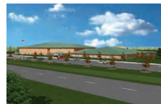
Figure 3-6 AFRC, Greenville, North Carolina
