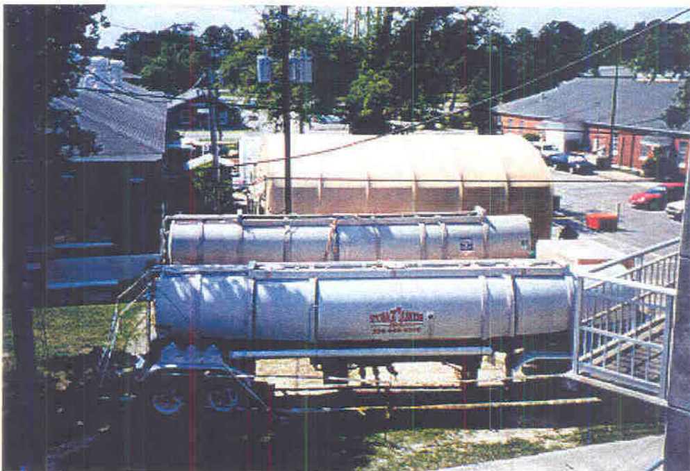
Wastewater tankers for disposal and for contingency
