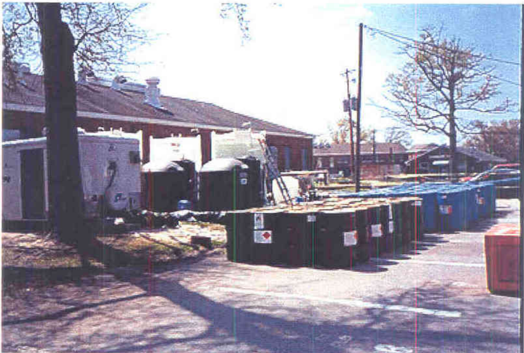
A view of the site facing southwest showing the calcium chloride tanks (black), isopropyl alcohol drums (black) and surfactant drums (blue)
