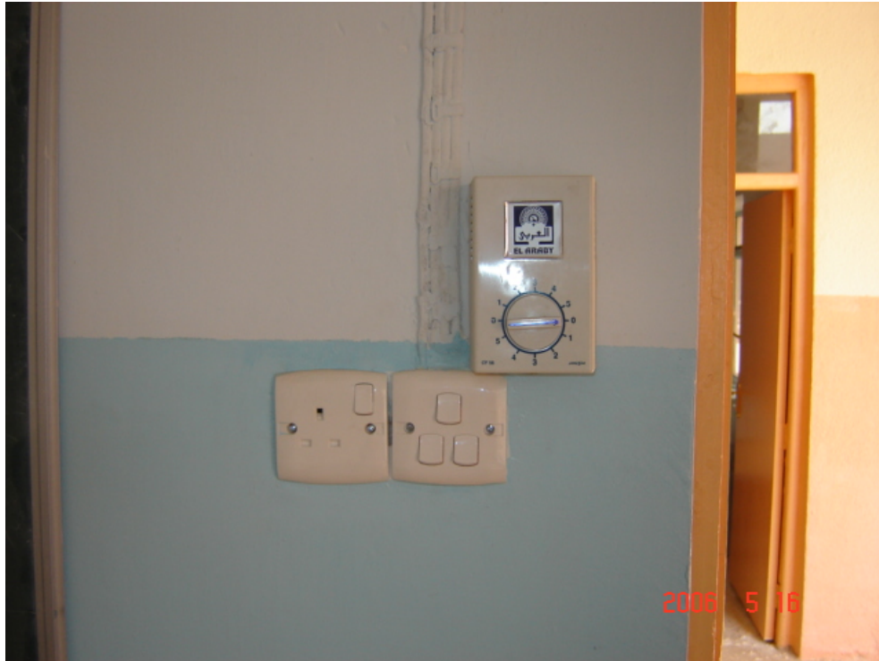
Site Photo 8. Correctly installed electrical switches and ceiling fan control after renovation (Photo courtesy of USACE)
