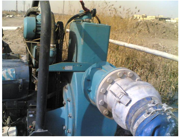
Site Photo 12. Diesel pump used at the manhole outside the G-7 lift station (Photo courtesy of USACE)
