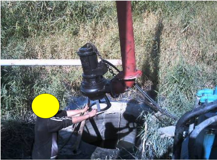
Site Photo 11. Installation of 150 mm submersible pump into manhole outside G-7 lift station (Photo courtesy of USACE)
