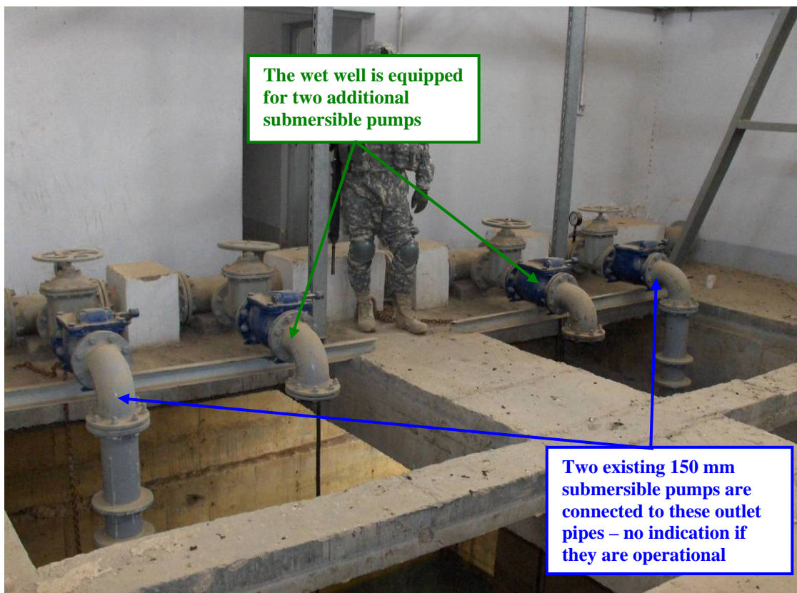
Site Photo 2. Interior view of Al Ghazaliyah G-7 Sewage Lift Station building
