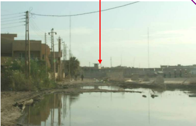
Site Photos 4 and 5. Backed-up sewer water in the Al Ghazaliyah area of Baghdad
