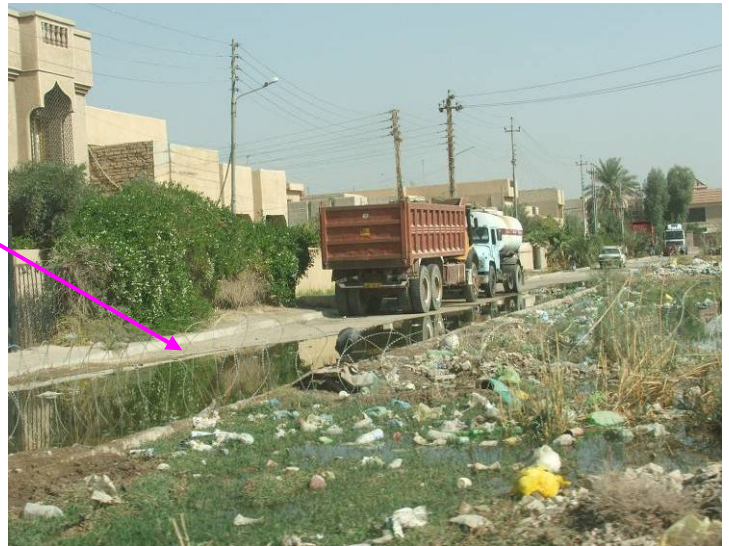
Site Photo 3. Backed-up sewer water
