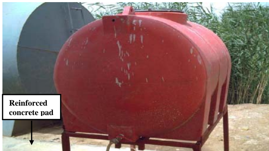
Site Photo 17. 1,000 liter generator fuel tank
