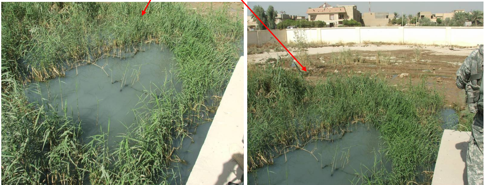
Site Photos 6 and 7. View of pool of accumulated sewage water outside the G-7 lift station
