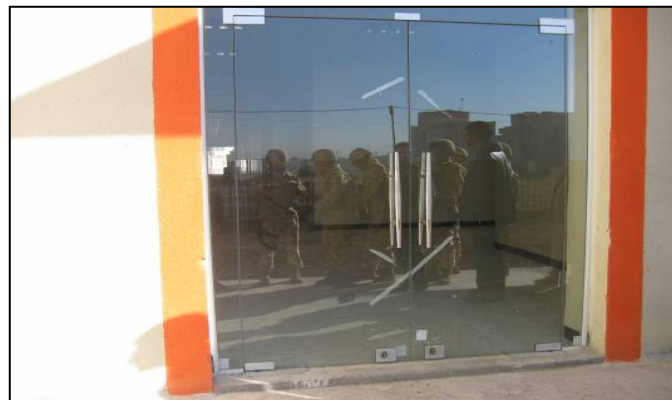
Site Photo 5. Tempered glass entry door
