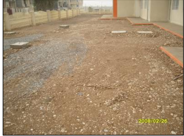
Site Photo 2. Correction of grading and grading level subsequent to site visit (Photo courtesy MND-NE).
