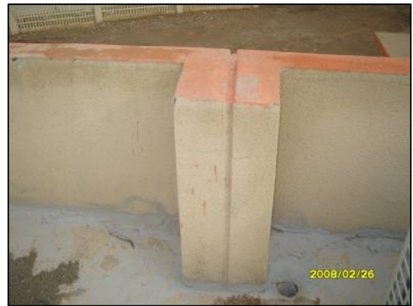
Site Photo 20. Corrective action subsequent to site visit to reconstruct parapet and expansion joint. (Photo courtesy of MND-NE).
