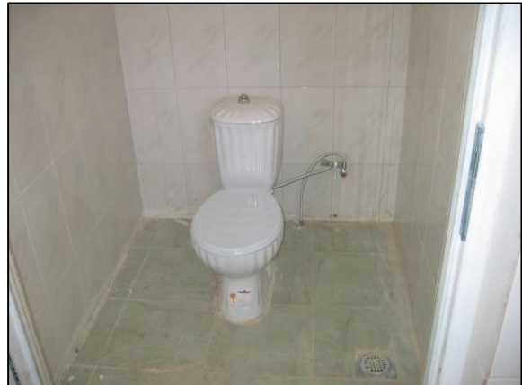
Site Photo 13. Western toilet
