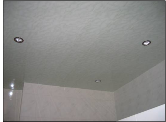
Site Photo 11. Bathroom ceiling
