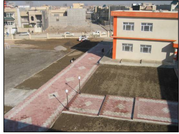
Site Photo 4. Outside building finish
