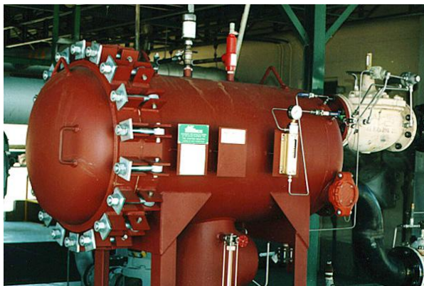
Figure 27. New Filter Separator Vessel
