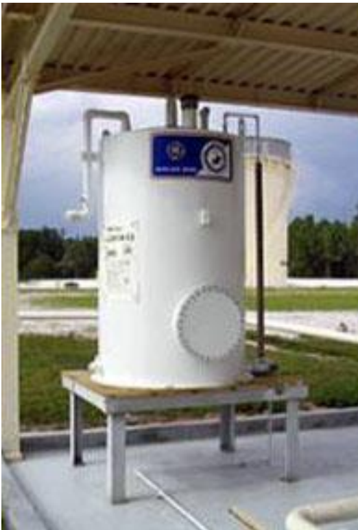
Figure 95. 500 Gallon (US) Bulk Additive Storage Tank
