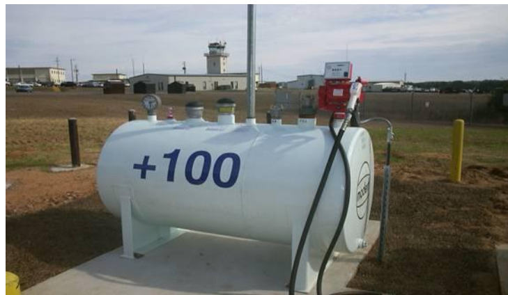
Figure 25. Bulk Storage of Neat Additive
