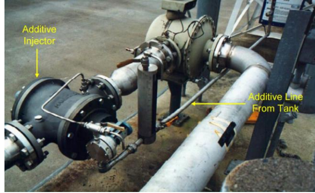
Figure 94. Additive In-Line Injector, Additive Feed and Fuel Line Connections
