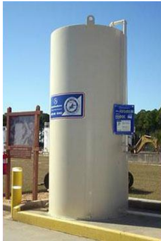
Figure 96. 2000 Gallon (US) Bulk Additive Storage Tank
