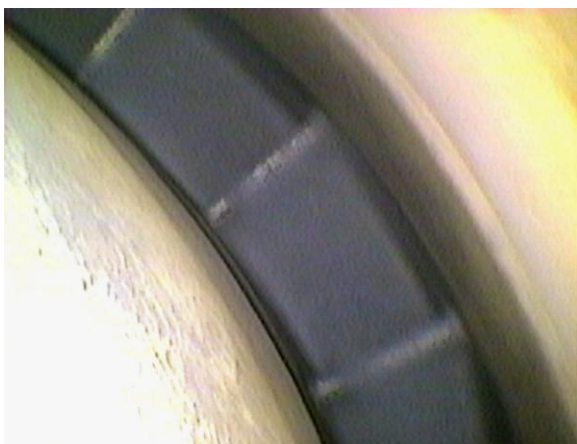
Figure 87. Baseline Condition of Exit Vanes
