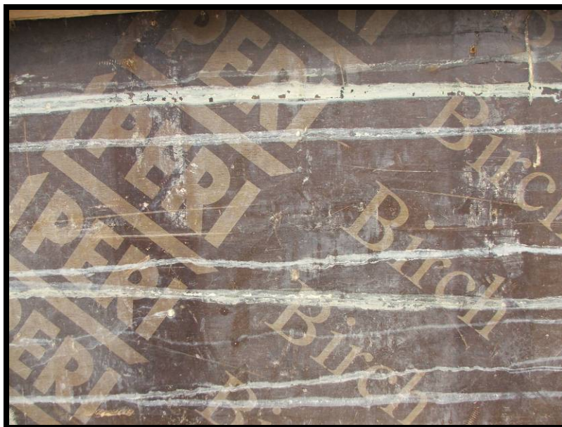
Site Photo 15. Contractor used premium forming materials.
