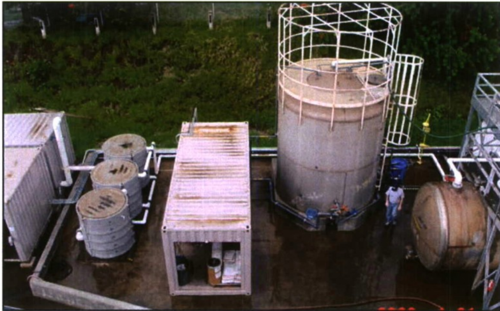
Figure 2. Oily Sludge Bioreactor at NAVSTA Pearl Harbor, HI. From left-to-right are the control room and blower facilities, biocubes, ultrafiltration module, reactor, and tanks for receiving sludge and storing ultrafiltrate permeate.
