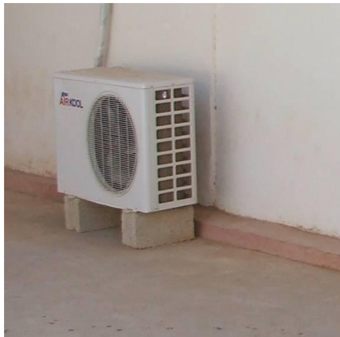
Site Photo 10. Split air-conditioning unit
