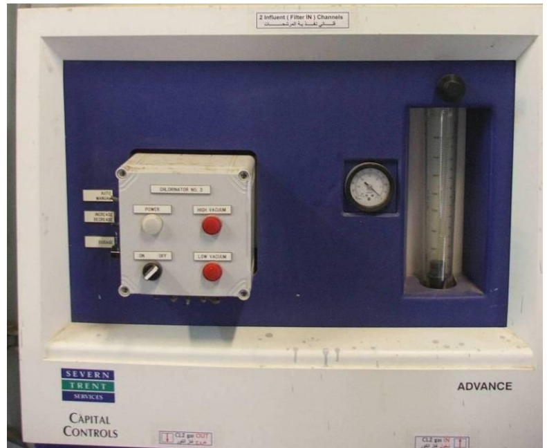
Site Photo 25. Remote chlorine injector
