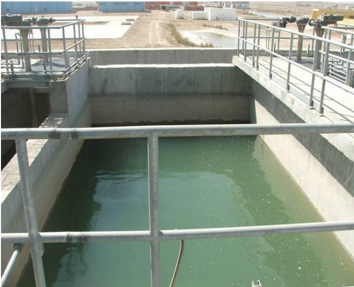
Site Photo 19. Filter tank
