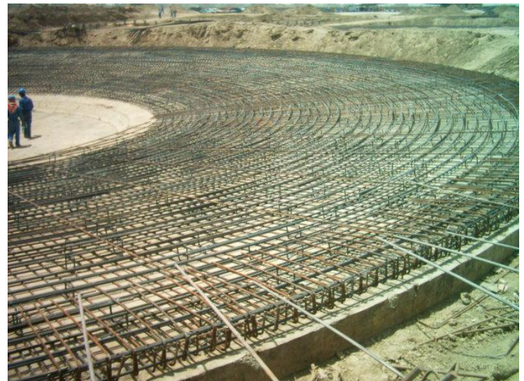
Site Photo 6. Steel reinforcement for clarifier base (Photo courtesy of the USACE)
