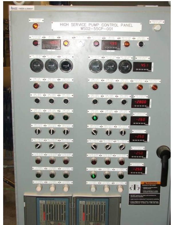
Site Photo 22. High service pump control panel
