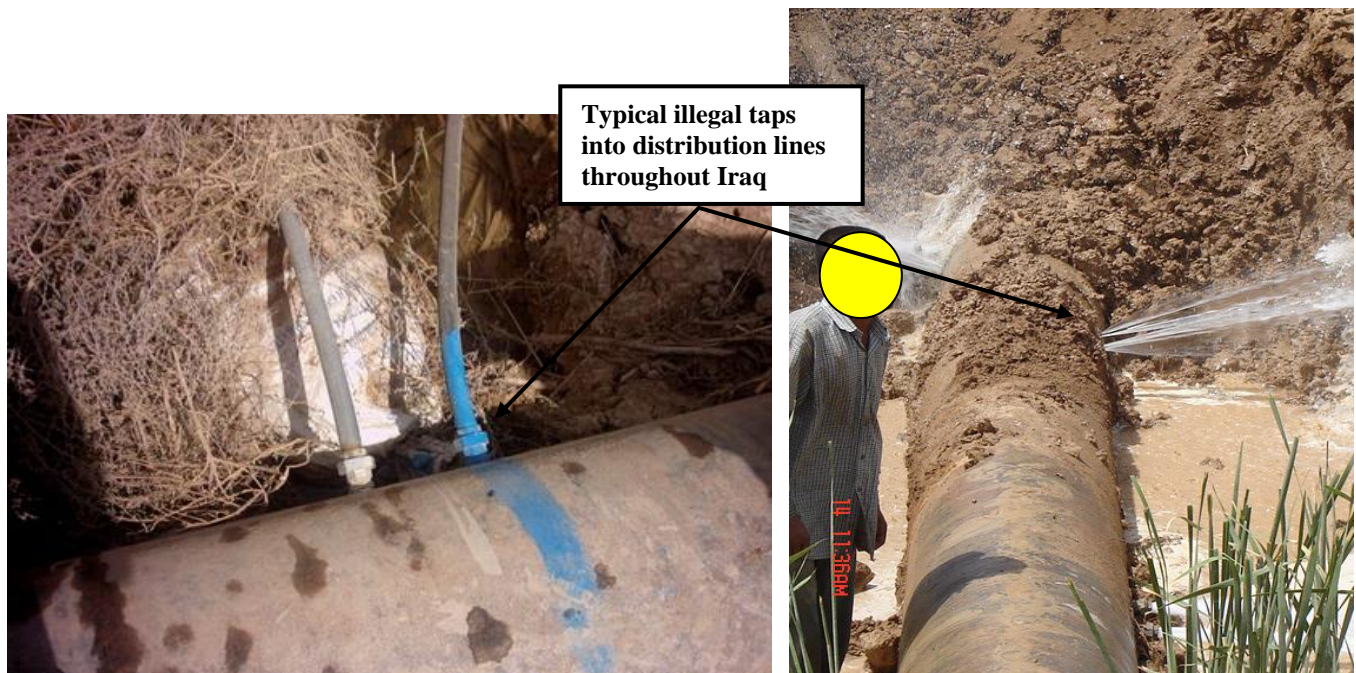
Site Photos 31 and 32. Examples of typical illegal taps and leaks in the distribution lines throughout Iraq
