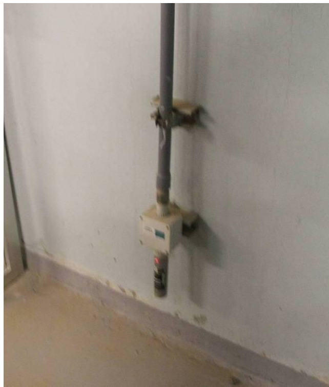
Site Photo 26. Chlorine leak detector
