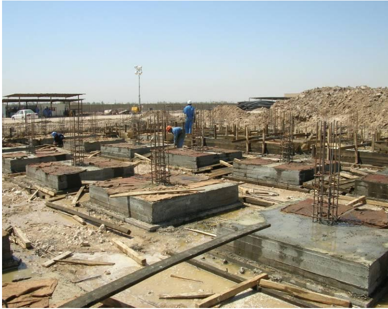
Site Photo 3. Concrete foundation for the chlorination area (Photo courtesy of the USACE)
