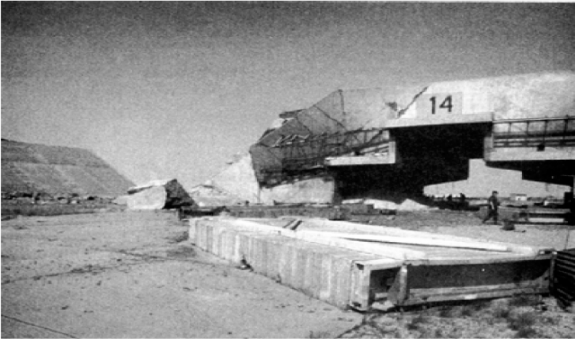
The Iraqi air force had essentially "hunkered down" to protect itself. The coalition undertook a major effort to find and destroy the sheltered aircraft so that the Iraqis could not use them later in a surprise "Tet-like" offensive. Here, steel blast doors from an aircraft shelter have been blown across the tarmac after a coalition air attack.
