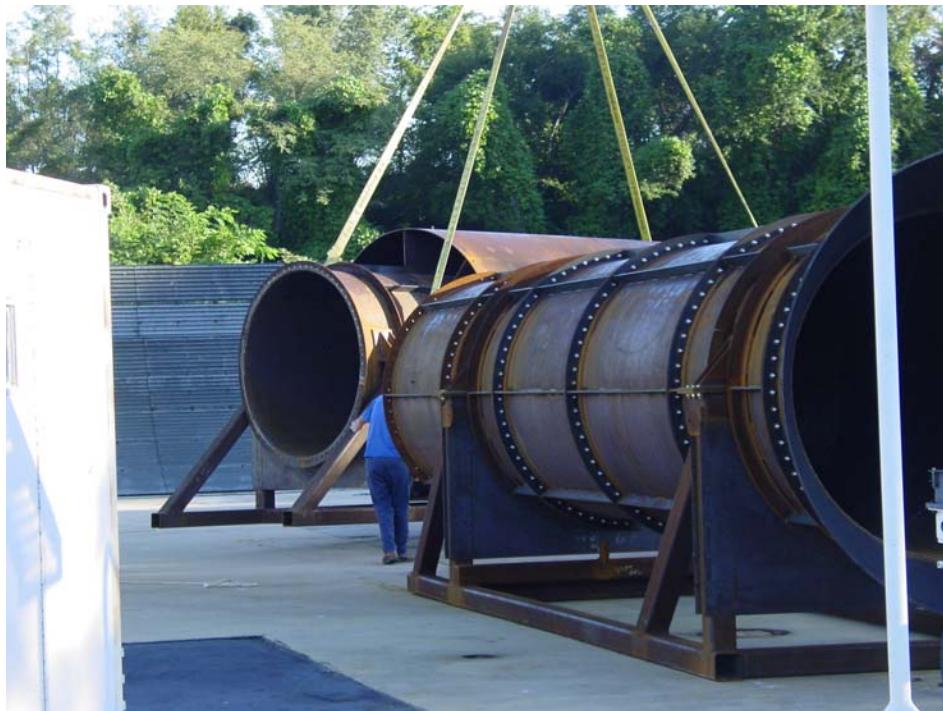
Figure 3.16 Crane Lifting Aft Section of NAD into Place.
