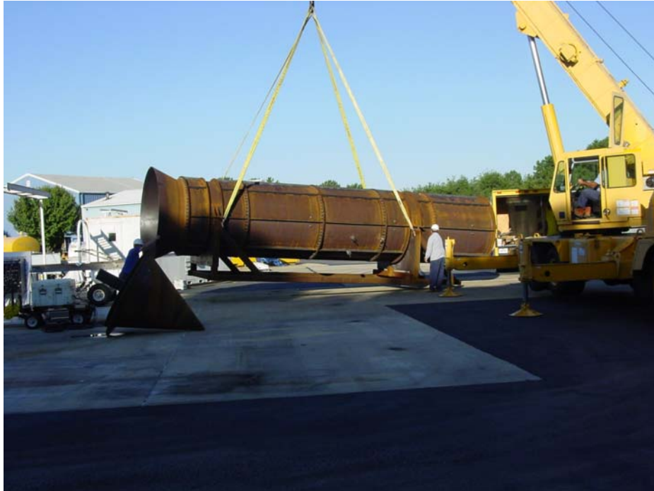
Figure 3.15 Crane Lifting Forward Section of NAD into Place.
