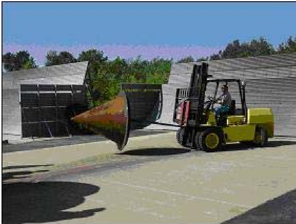
Figure 3.18 Moving Exhaust Cone (NADc) into Place for Attaching to NADc.
