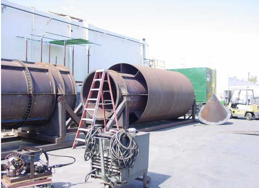
Figure 3.8 NAD During Fabrication at GE-EER Plant in Santa Ana, California.
