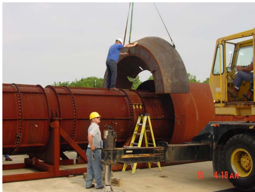
Figure 4.9 Installing Top Central Piece of Flow Deflector.
