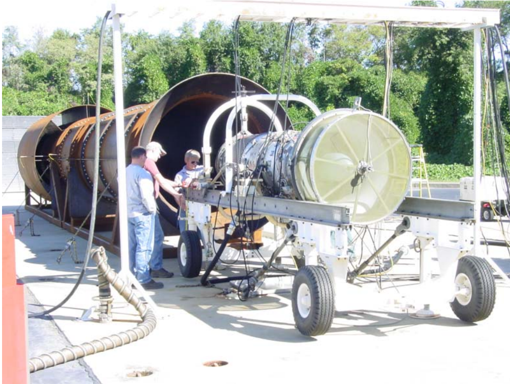
Figure 3.25 Making Final Adjustments on J-52 Engine Installation.
