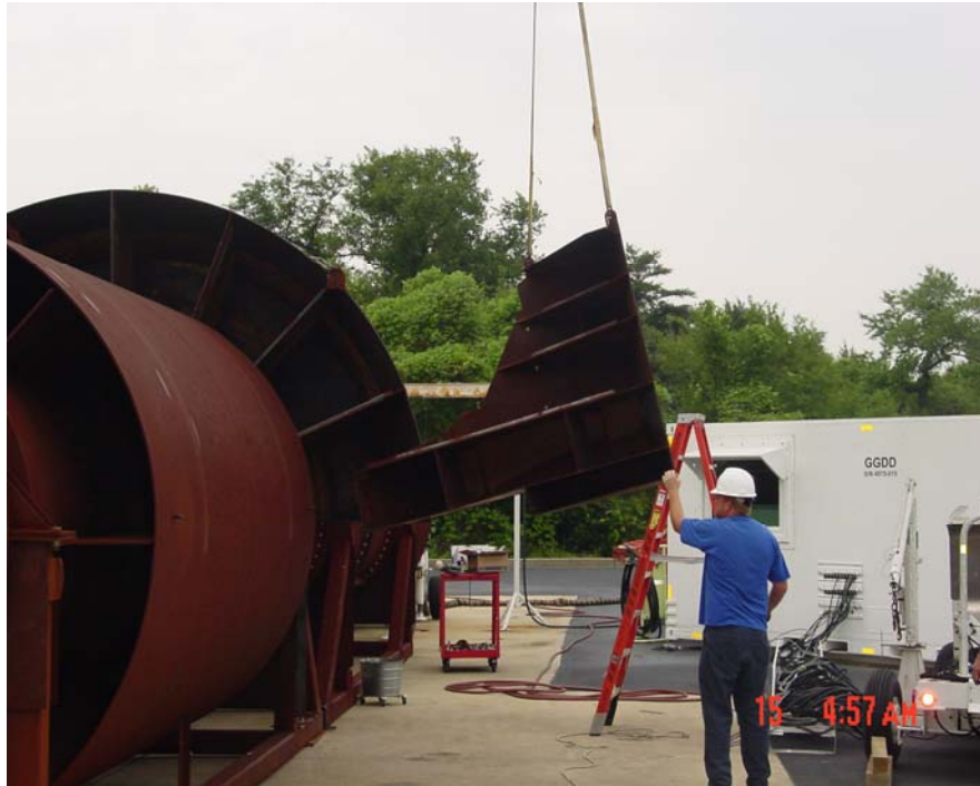
Figure 4.10 Installing Lower Side Piece of Flow Deflector.
