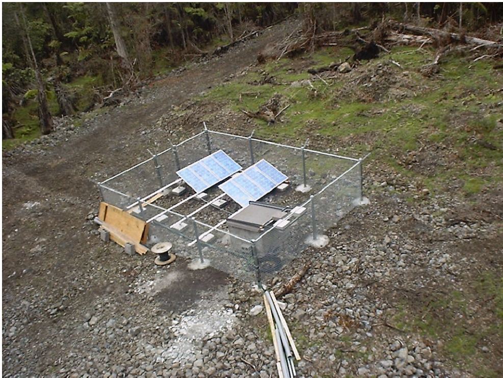
Figure 7. Central photovoltaic power system.
