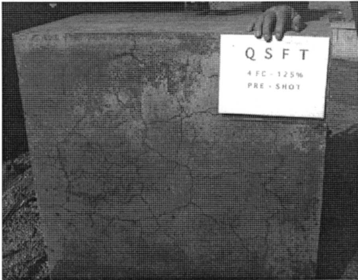
Figure 13. Visible cracking on the bottom of the floor section block while it was hoisted on its side for inspection.
